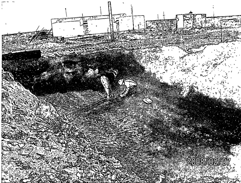
COMPACTION OF INSTALLED CLAY BEING MEASURED
