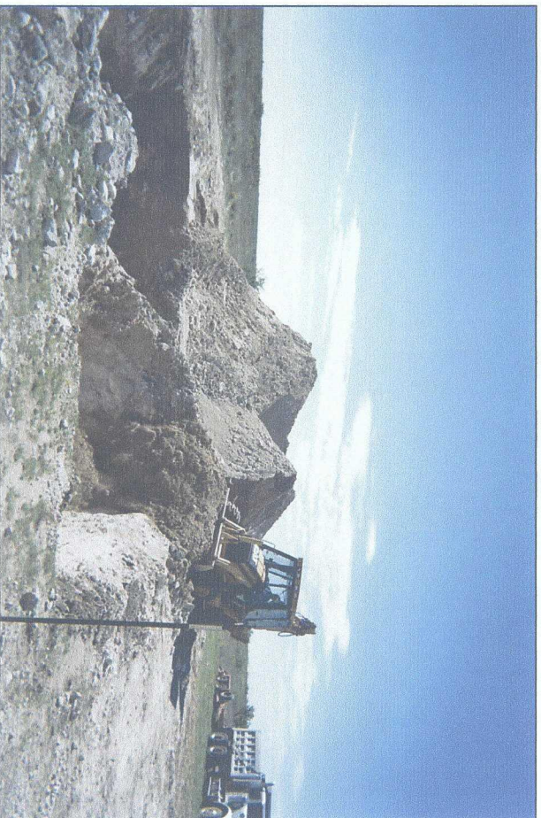
backfilling excavation
