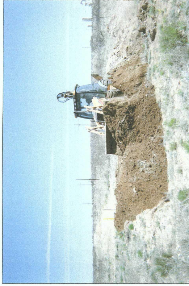
backfilling with clean, imported backfill
