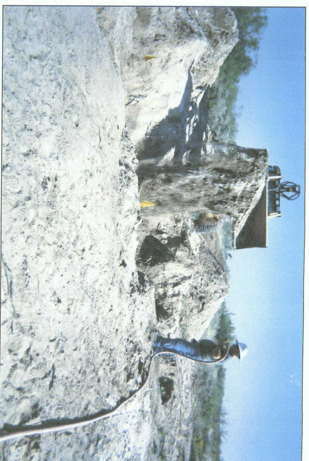
backfilling delineation trenches
