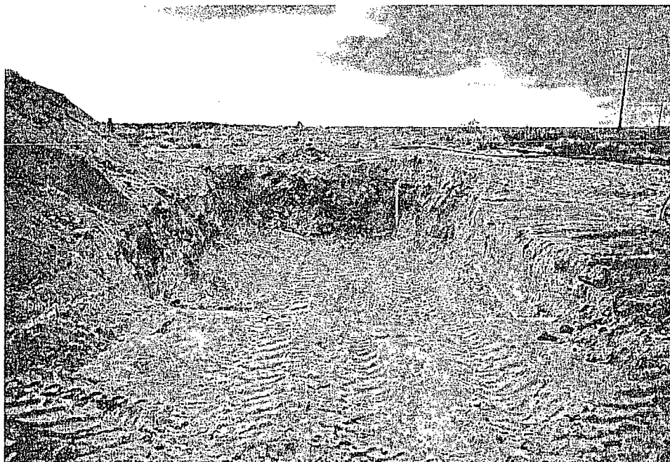
Figure 4: Preparation for installation of ET barrier
