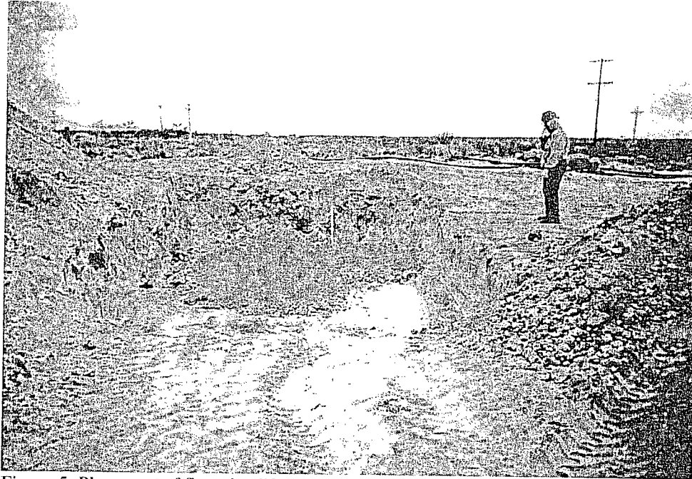
Figure 5: Placement of first clay lift on prepared surface
