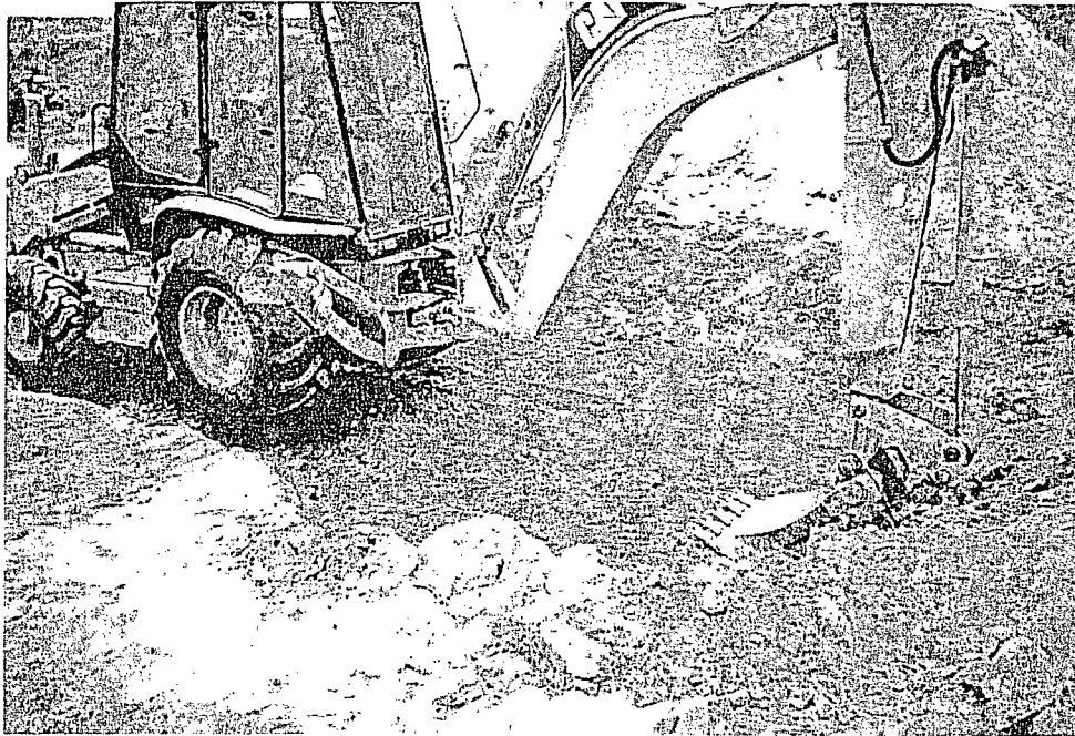
Figure 7: Compaction of clay layer
