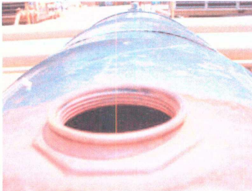
Photo 28: Saddle tank missing bung, two of three tanks missing lid.
