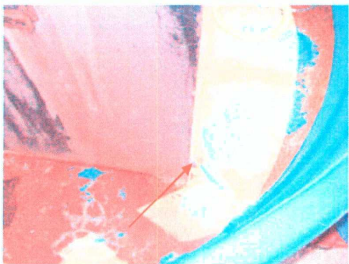
Photo 9 : Arrow shows the used oil filter secondary containment plug.
