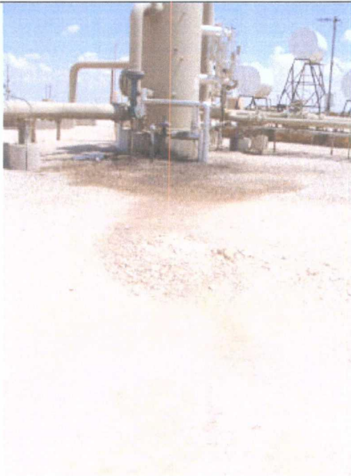
Photo 27: Discharge on ground from sulfur unit, allowed to drain.
