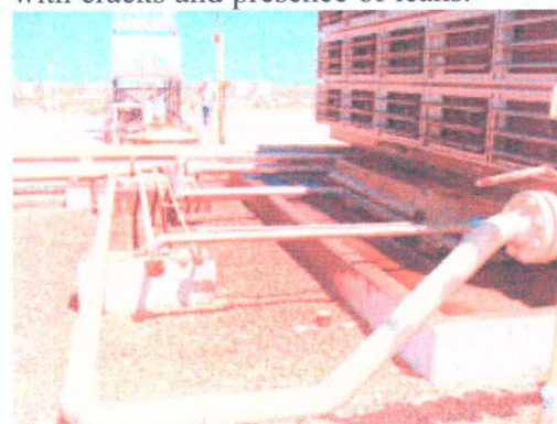
Photo 16: Gravel soiled around compressor.
