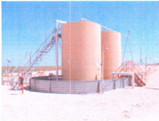
Photo 1 : Two AST's with secondary containment.
