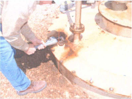
Photo 19: Leak detection being removed using a tool.
