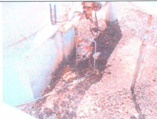
Photo 25 : Sulfur unit with discharge on to ground.
