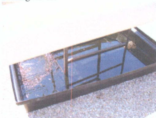
Photo 23 : Another secondary containment full of fluids.
