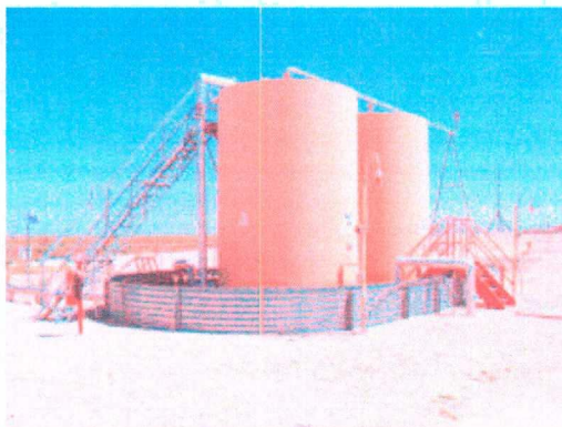
Photo 1: Two AST's with secondary containment.
