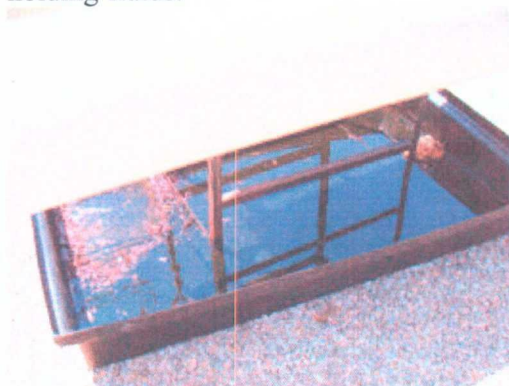
Photo 23 : Another secondary containment full of fluids.
