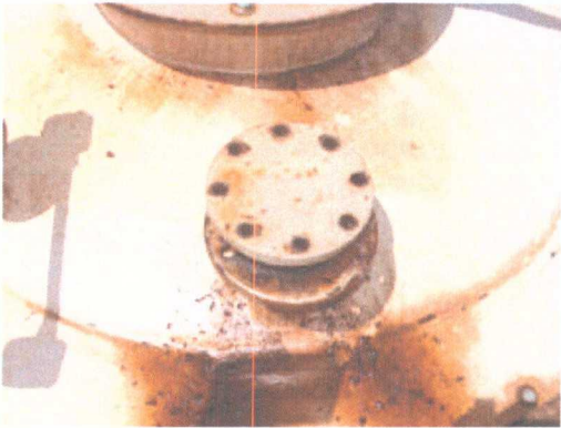
Photo 18: Flange resting over port above BGT. Pressurized, flow of "air".
