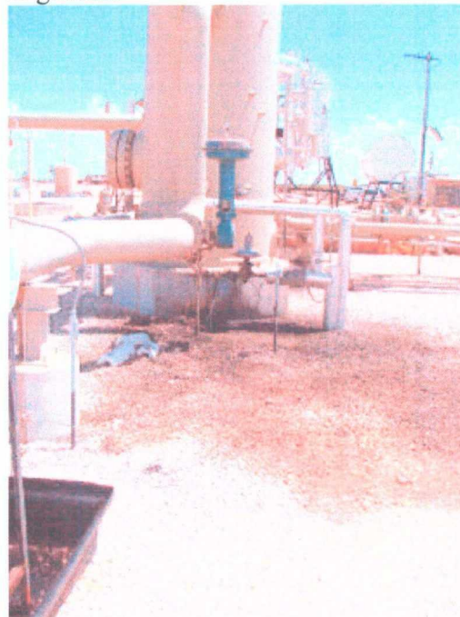
Photo 26 : Sulfur unit with discharge on ground.
