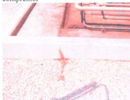
Photo 15: A secondary containment area with cracks and presence of leaks.
