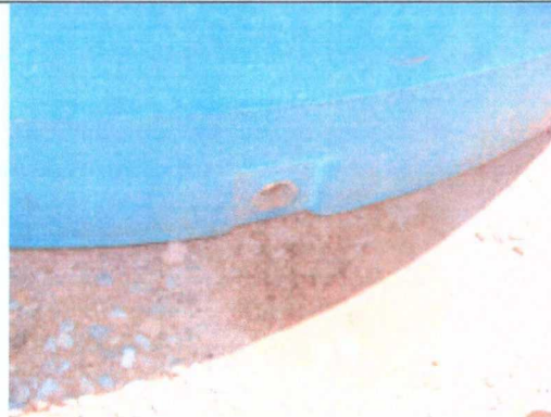
Photo 10: Third containment barrier for used filter holding area missing its bung, with discharge on to the ground.
