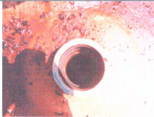
Photo 20: Fluids are present in leak detection system.
