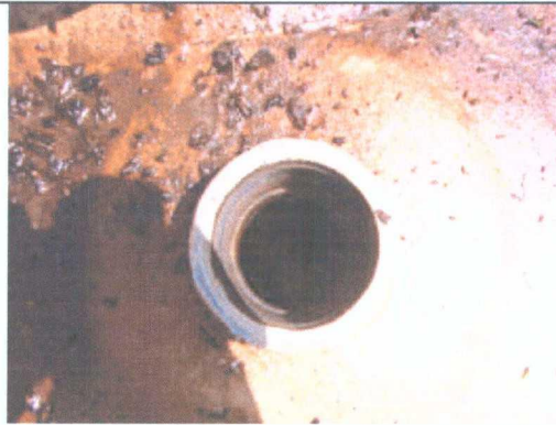
Photo 20: Fluids are present in leak detection system.
