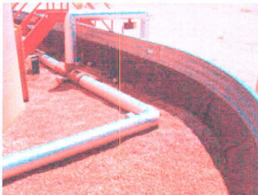
Photo 2: discharge within the secondary containment area
