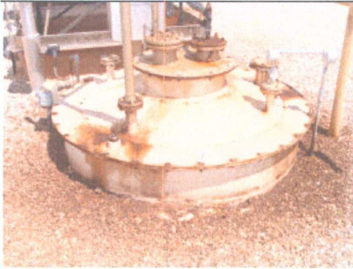
Photo 17: BGT with discharge around its area.
