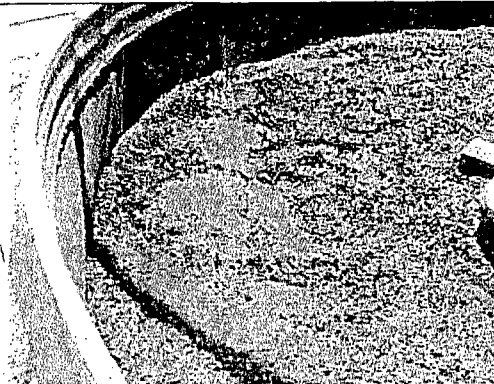
Photo 4 : Free liquids in secondary containment.
