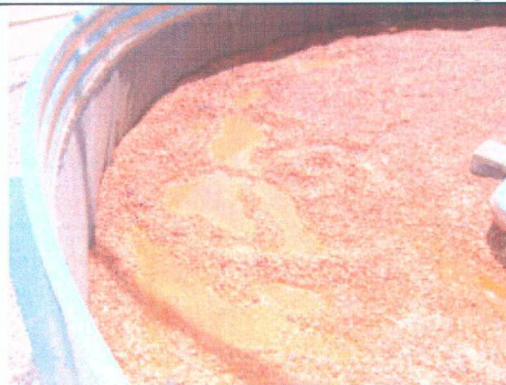
Photo 4 : Free liquids in secondary containment.
