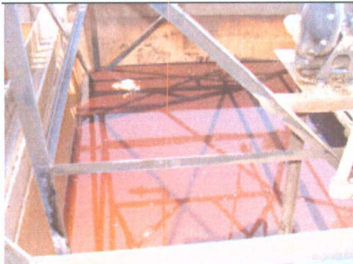
Photo 22 : Secondary containment holding fluids.
