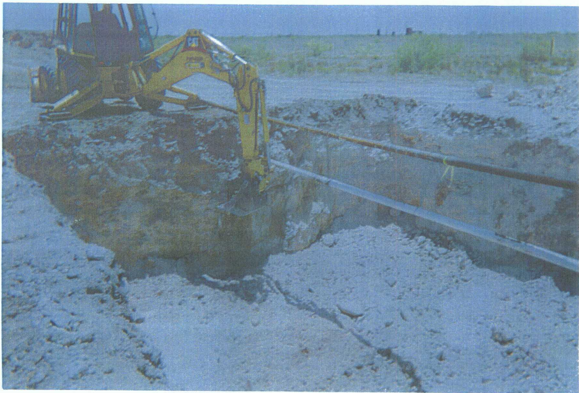
6. Excavation of soils around junction box.
