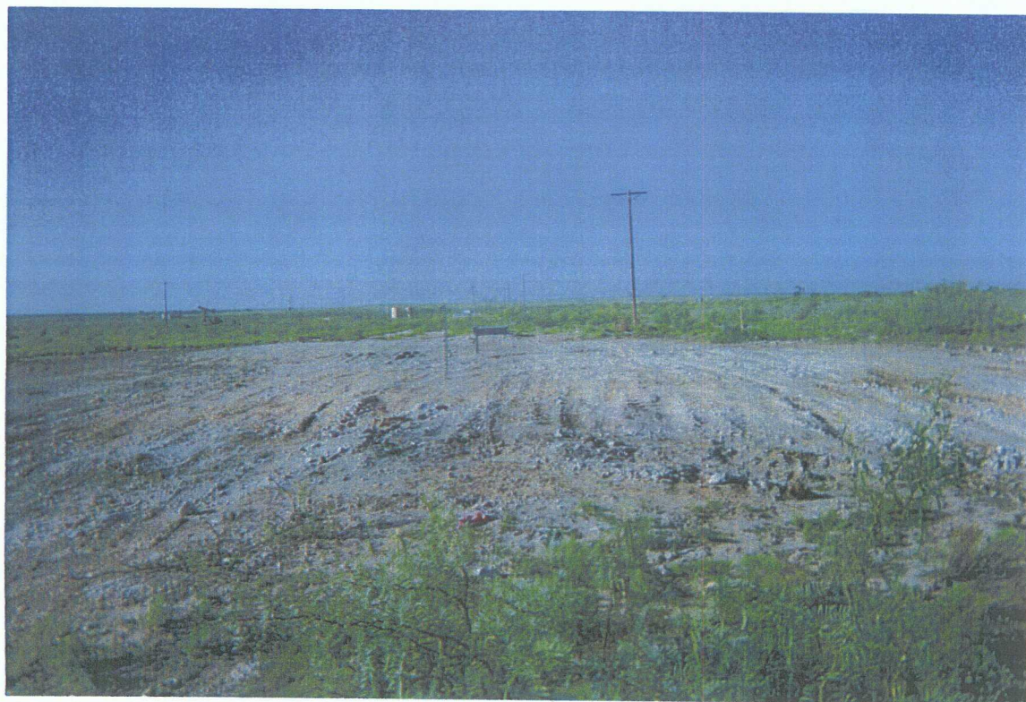
8. Completed backfilling of soils around junction box.
