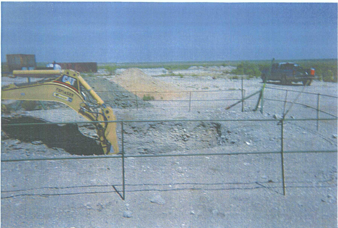
4. Excavation of soils around junction box.
