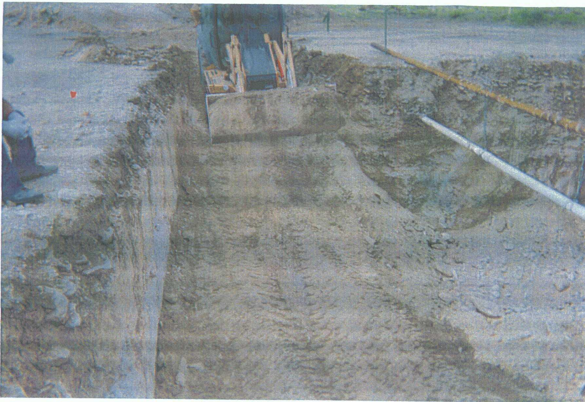
7. Backfilling of soils around junction box.
