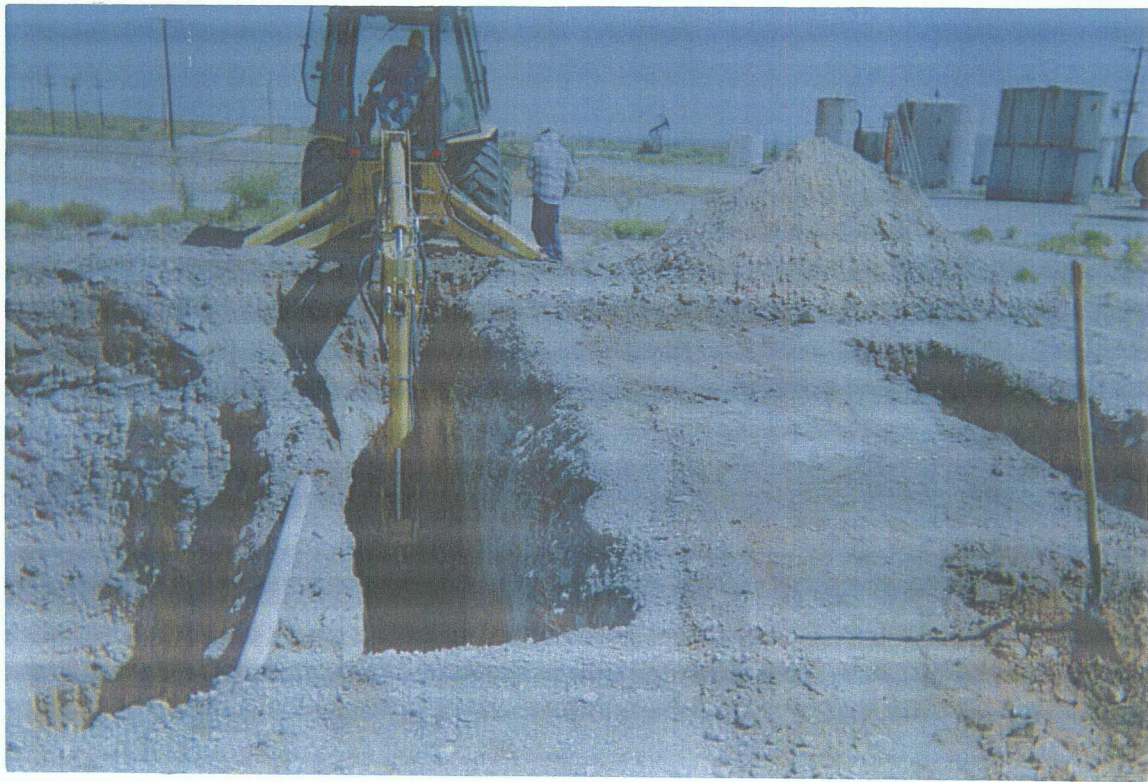
5. Excavation of soils around junction box.
