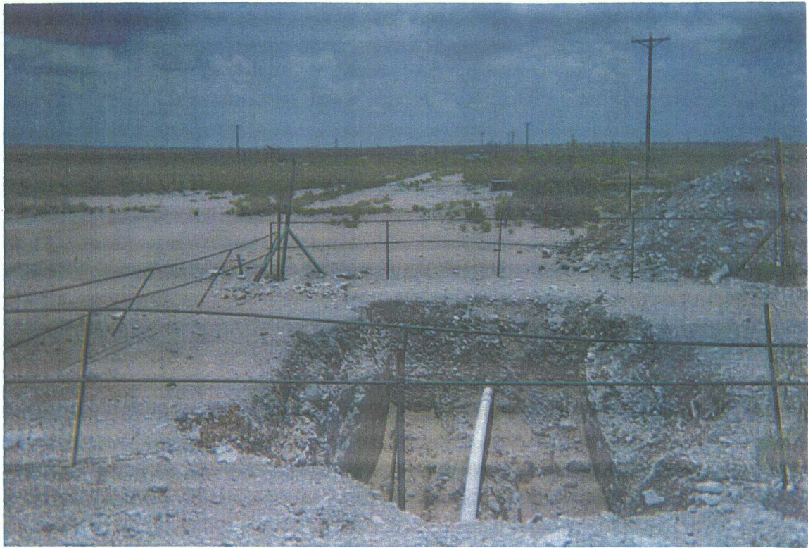
3. Excavation of soils around junction box.
