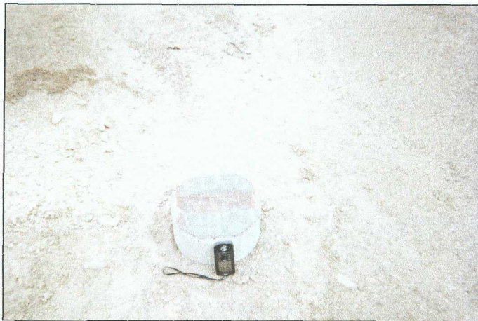
Identification plate to mark former junction site and clay barrier below.
