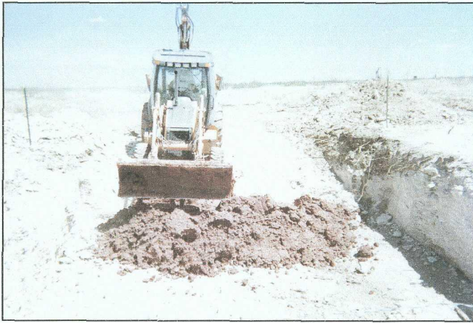
Installing clay barrier at 6 ft: 4/13/2006
