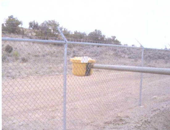
Photo 2: Catch pan installed on line.
