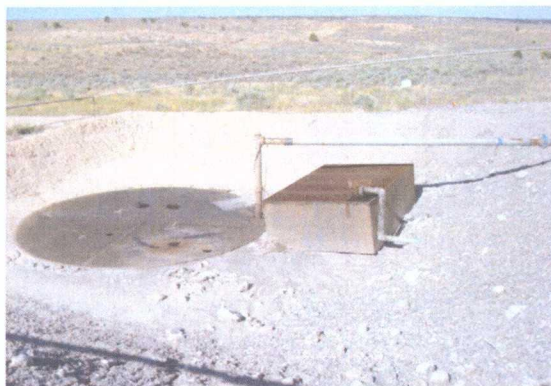
Photo 3: BGT removed from service.
