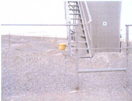
Photo 1: Catch pan installed on shortened load line.
