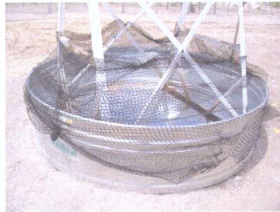
Photo 5: Secondary containment has been replaced.
