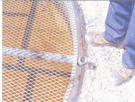
Image 9: Cap is missing and not in place of leak detection BGT.
