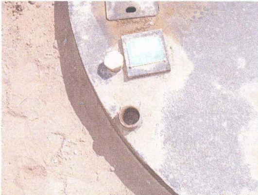
Image 2: Leak detection of questionable BGT has fluids.
