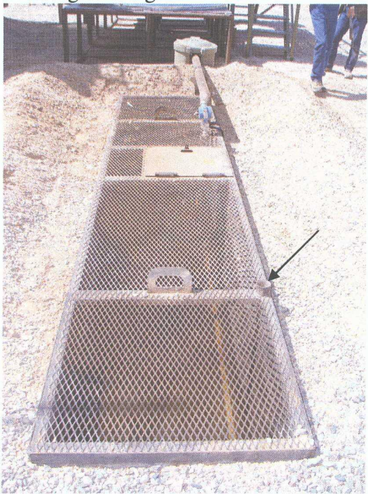
Image 8: Below grade catch tank is not identified on Lat. # 4 lay out schematic. The cap for the leak detector appears to be missing.
