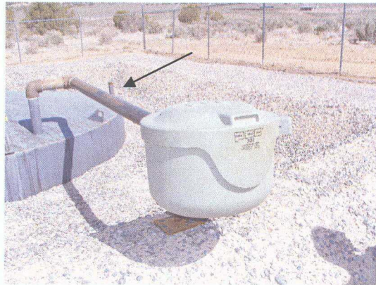
Image 10: Leak detection cap missing on sump located near entrance of facility.
