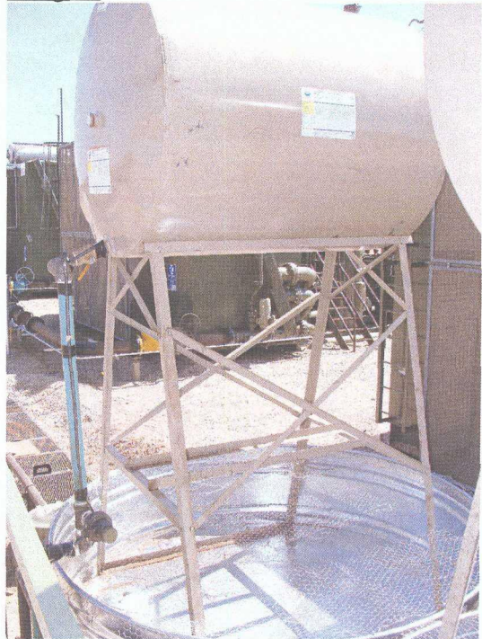
Image 6: Lube tank is bulged.
