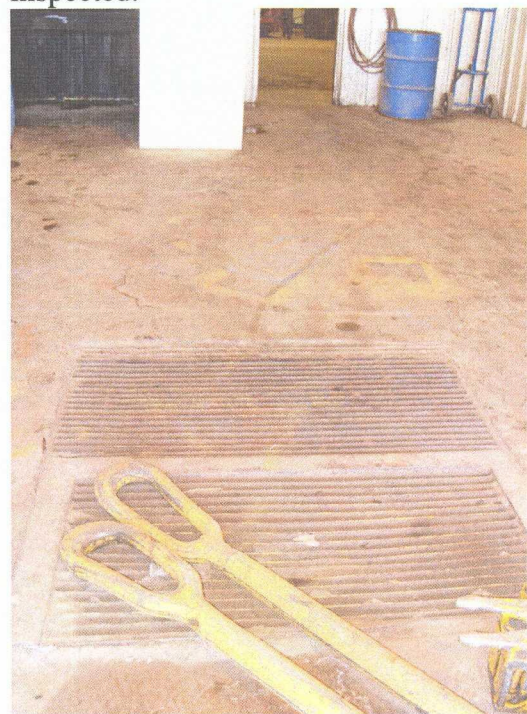
Photo 5: Sump with skimmer needs to be tested and inspected annually.
