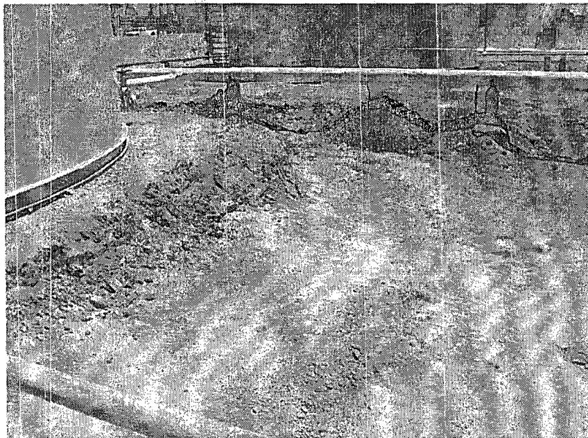
Figure 4: Excavation of contaminated soil in the area described in Figure 2. Note active pipeline towards the rear.
