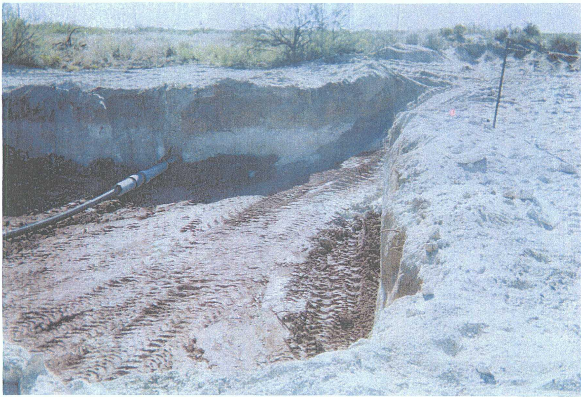
7. Clay liner at 6 feet bgs in excavation.
