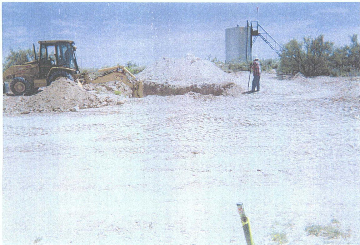
3. Excavation of soils around junction box.
