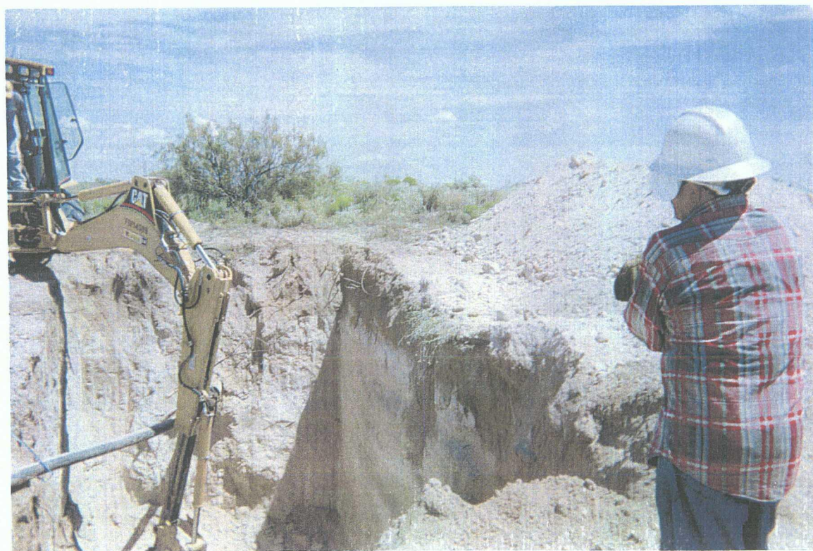
2. Excavation of soils around junction box.
