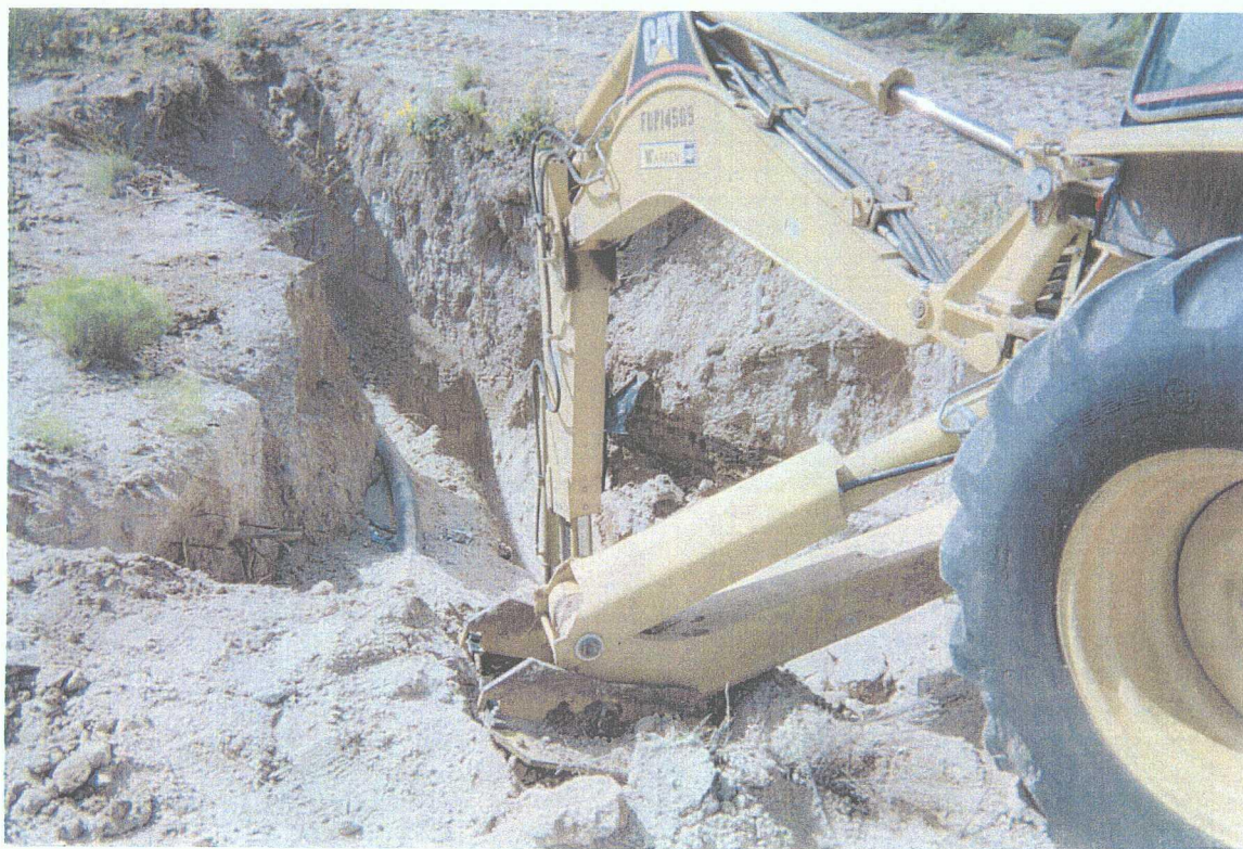
5. Excavation of soils around junction box.
