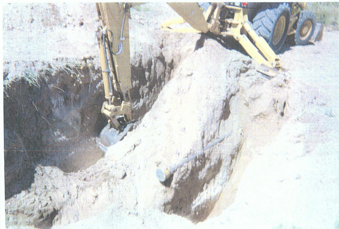
4. Excavation of soils around junction box.
