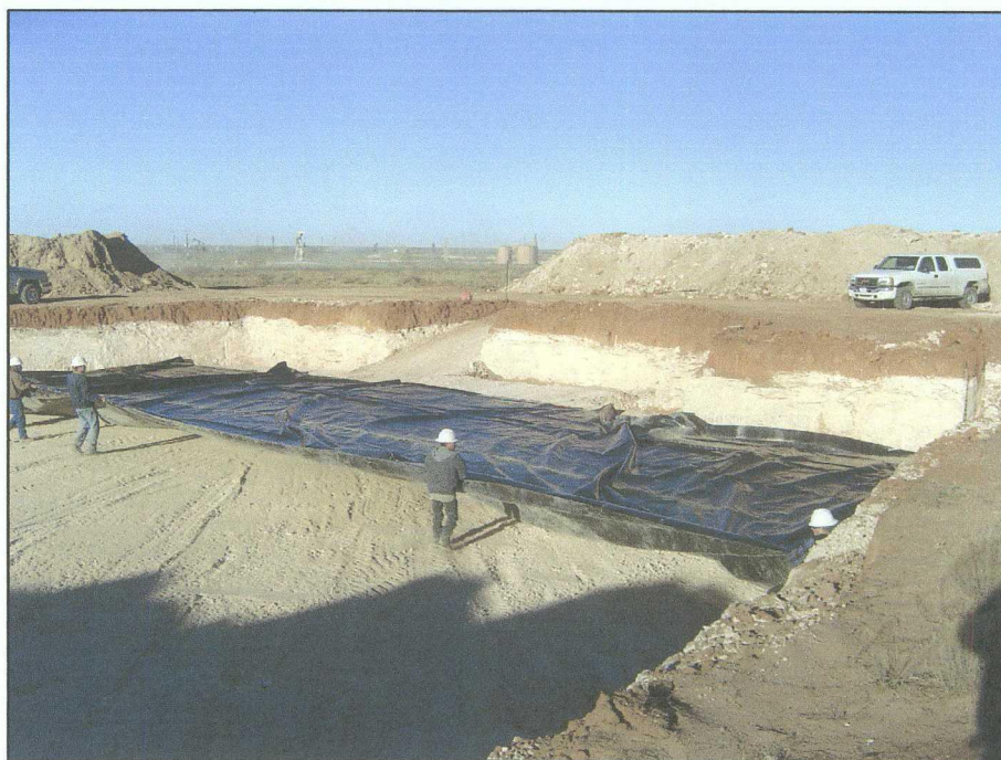
14. Pit Excavation Liner Installation Looking Southwest, February 19, 2008.
