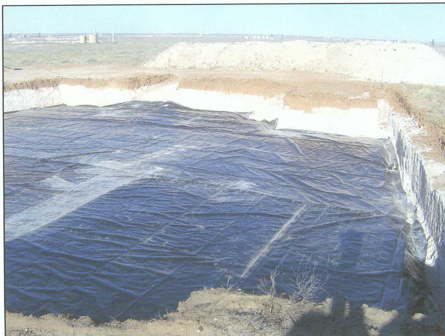
16. Pit Excavation Liner Installation Looking West, January 28, 2008.
