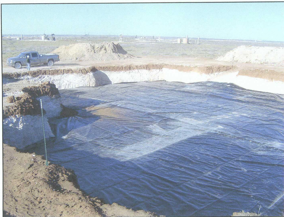
15. Pit Excavation Liner Installation Looking Southwest, January 28, 2008.
