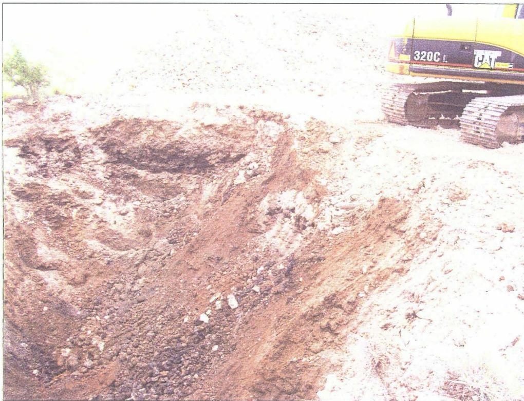
*No. 6 – View to the west of the excavation. Contamination is visible to the north and west, and clean fill material is piled to the west in the background.*
