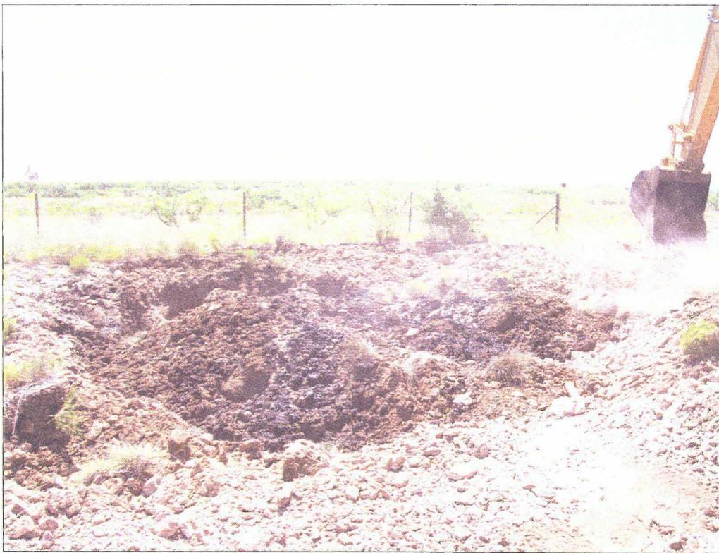
*No. 4 – View to the southeast of the excavation after mixing sludge with clean berm material to facilitate transport off Site.*
