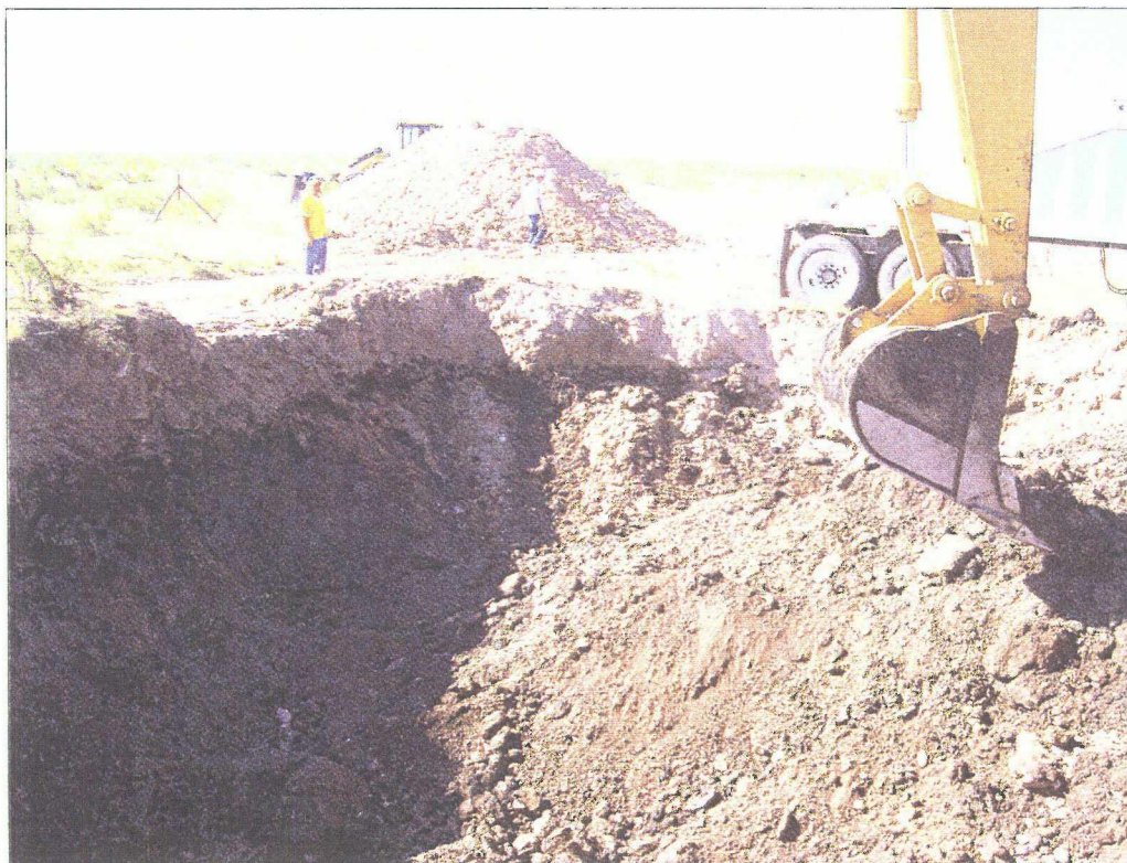
No. 4 – View of the south side of the pit showing extensive oil seepage (clean fill material is visible in the background).
