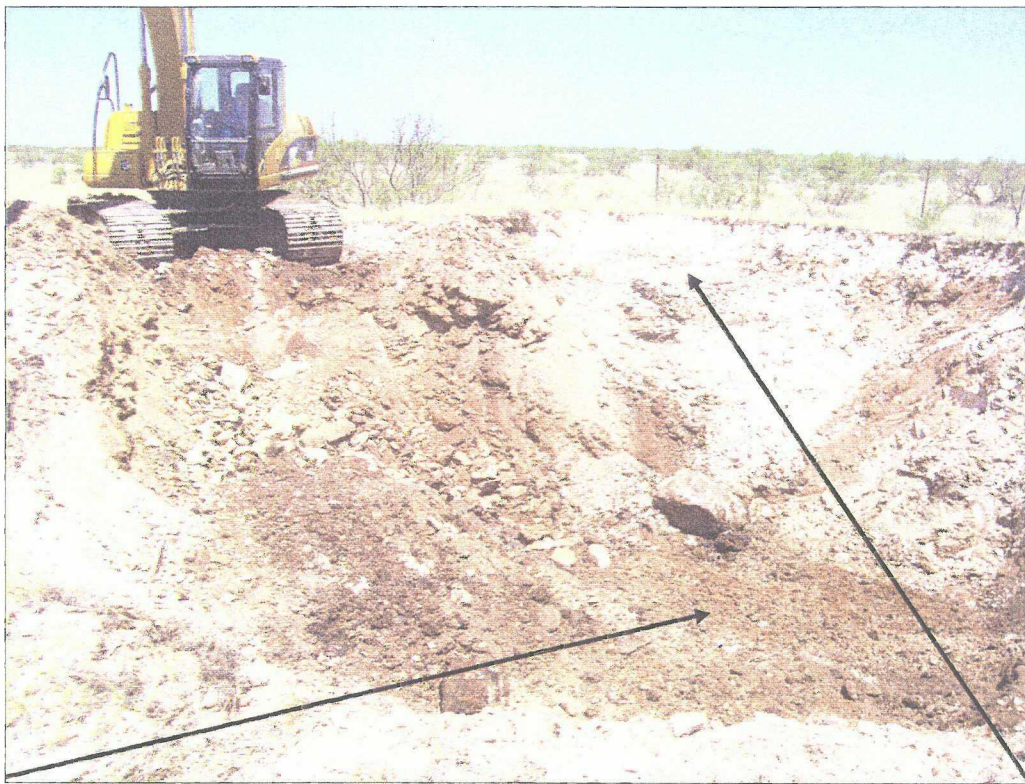
No 5 – View of the north and west ends of the pit showing what appears to be two clean ends of the pit (view is to the north/northwest). The impenetrable layer of caliche is highlighted with arrows.
