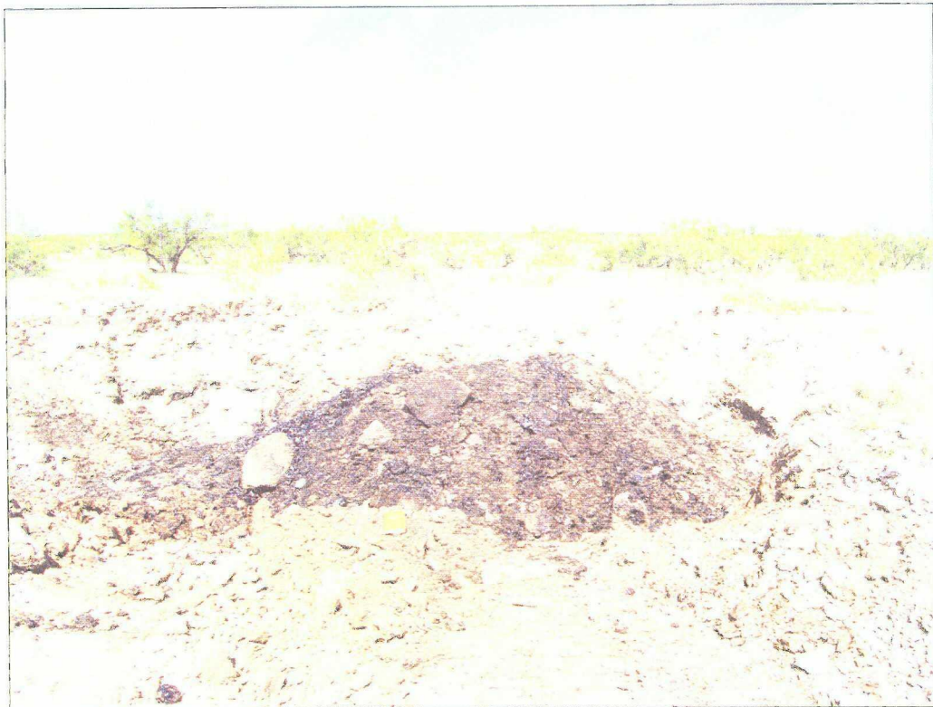
No. 2 – Pit material after mixing with clean berm material to facilitate transport off Site.
