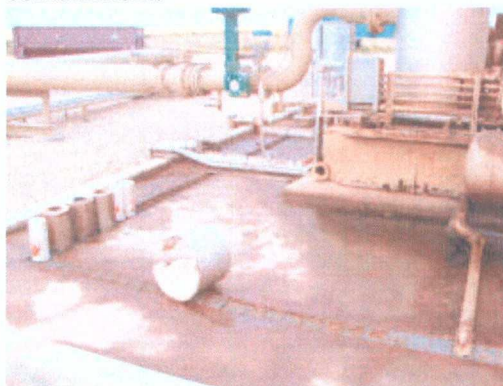
Photo 11 : Compressor skid with draining filters.
