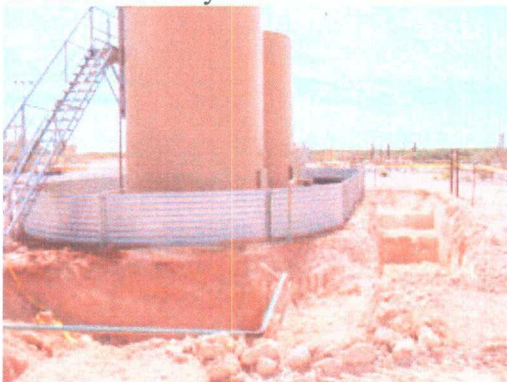
Photo 2: Excavation of spill on north and east side of tank batteries.
