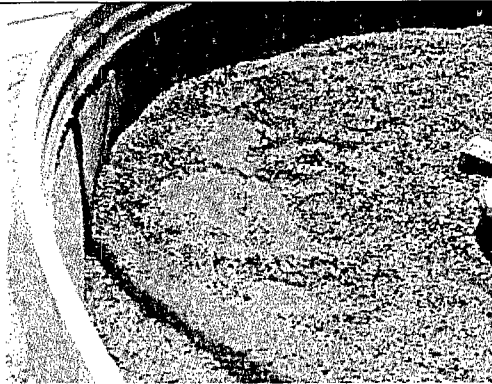
Photo 4: Free liquids in secondary containment.
