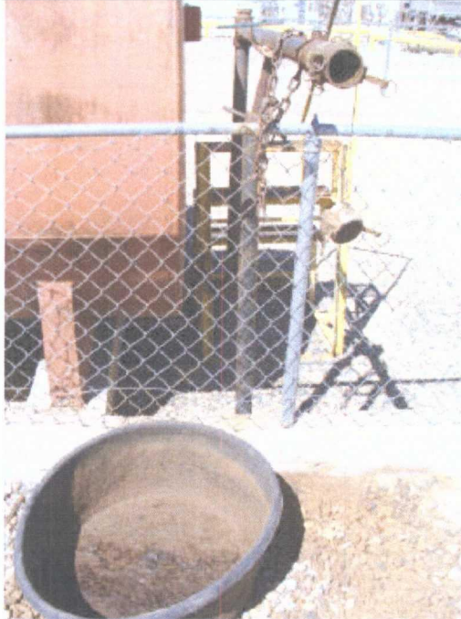
Photo 21: Drip pan area for used oil tank has discharge on to ground.
