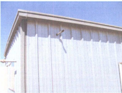
Photo 18: Conduit protruding from main fire pump building appears to have leaked diesel.
