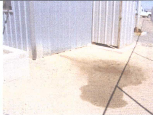
Photo 19: Leaked diesel on to ground underneath conduit of Photo 18.
