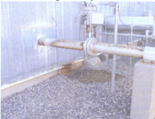
Photo 18: A leak at building and conduit interface.
