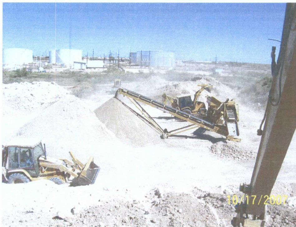
Frisco Skelly #1 – Screening activities prior to 40-mil poly liner installation
