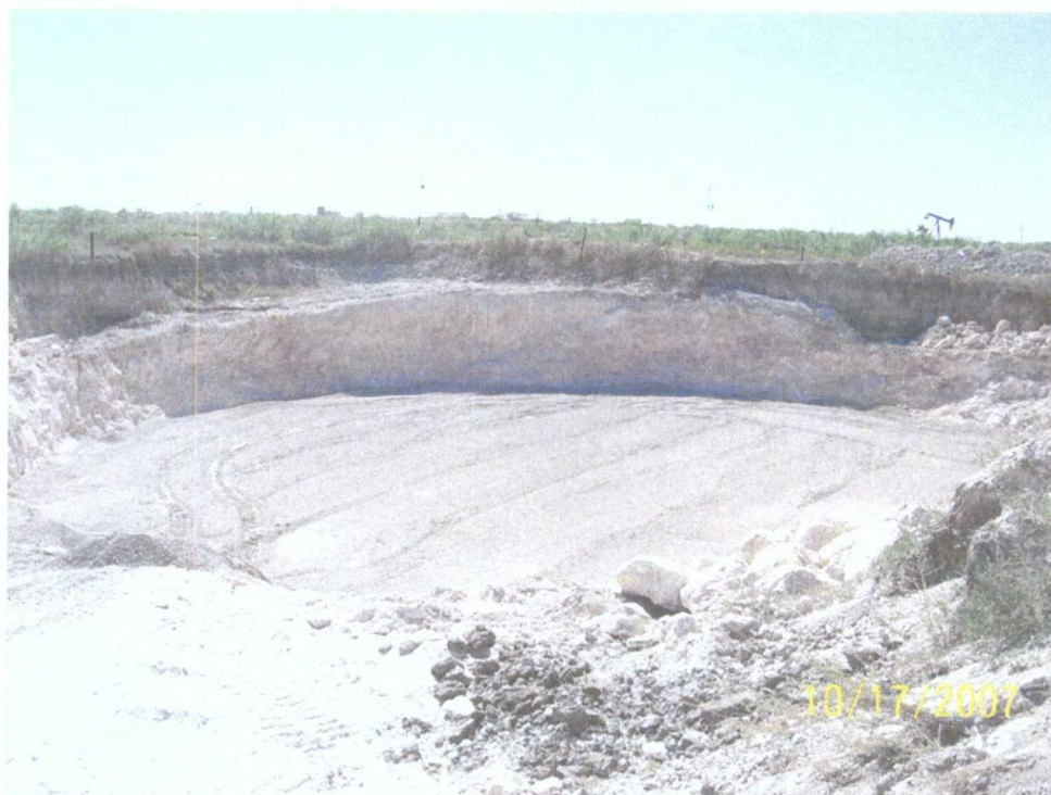
Frisco Skelly #1 – Lower layer of cushioning soil prior to liner installation
