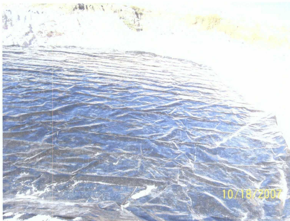
Frisco Skelly #1 – 40-mil poly liner installation
