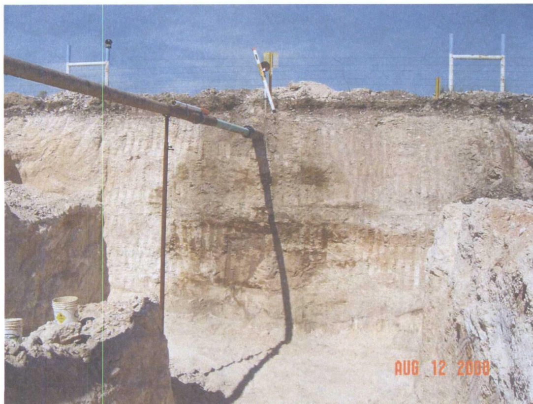
Photograph 6: The pit was over-excavated an additional 5 feet beyond the depth of residual affected soil at the base of excavation, as required prior to placement of the impermeable clay liner.
