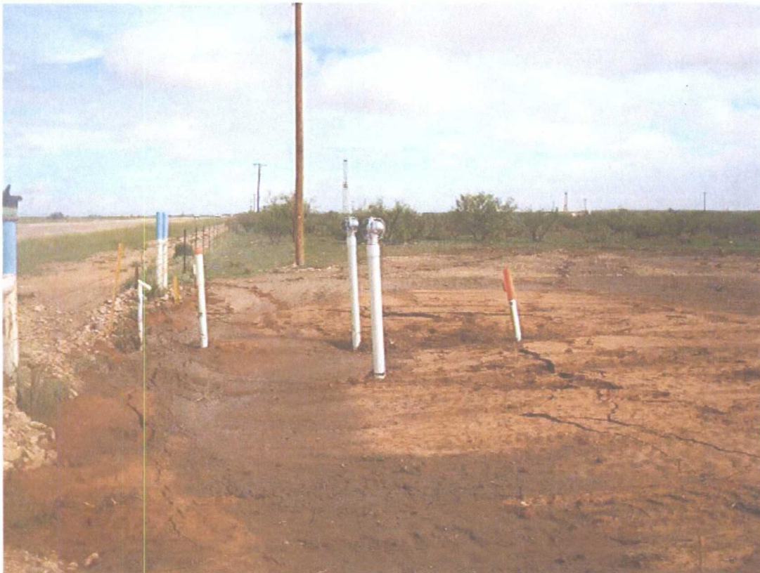
Photograph 14: Three feet of riser was left above the ground surface and 8-inch diameter wind turbines were permanently affixed to the 4" PVC riser.
