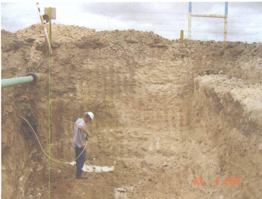
Photograph 10: The Micro-Blaze mixture was injected using 3,300 pounds per square inch of pressure into the affected sidewalls to a horizontal depth of at least 5-feet on 5-foot horizontal and 3-foot vertical centers.
