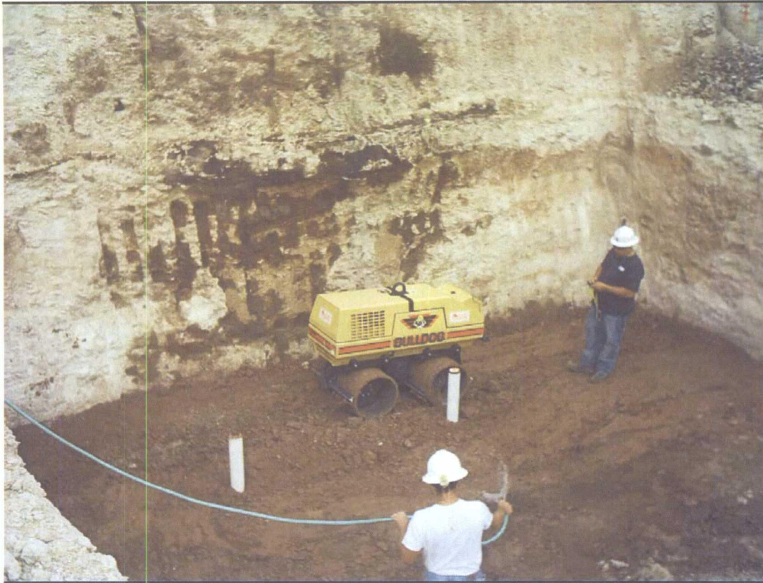
Photograph 11: The 2-foot thick clay barrier was installed in 6-8 inch lifts and compacted down to 4 to 5 inches using a 36 inch wide, ride on roller compactor.
