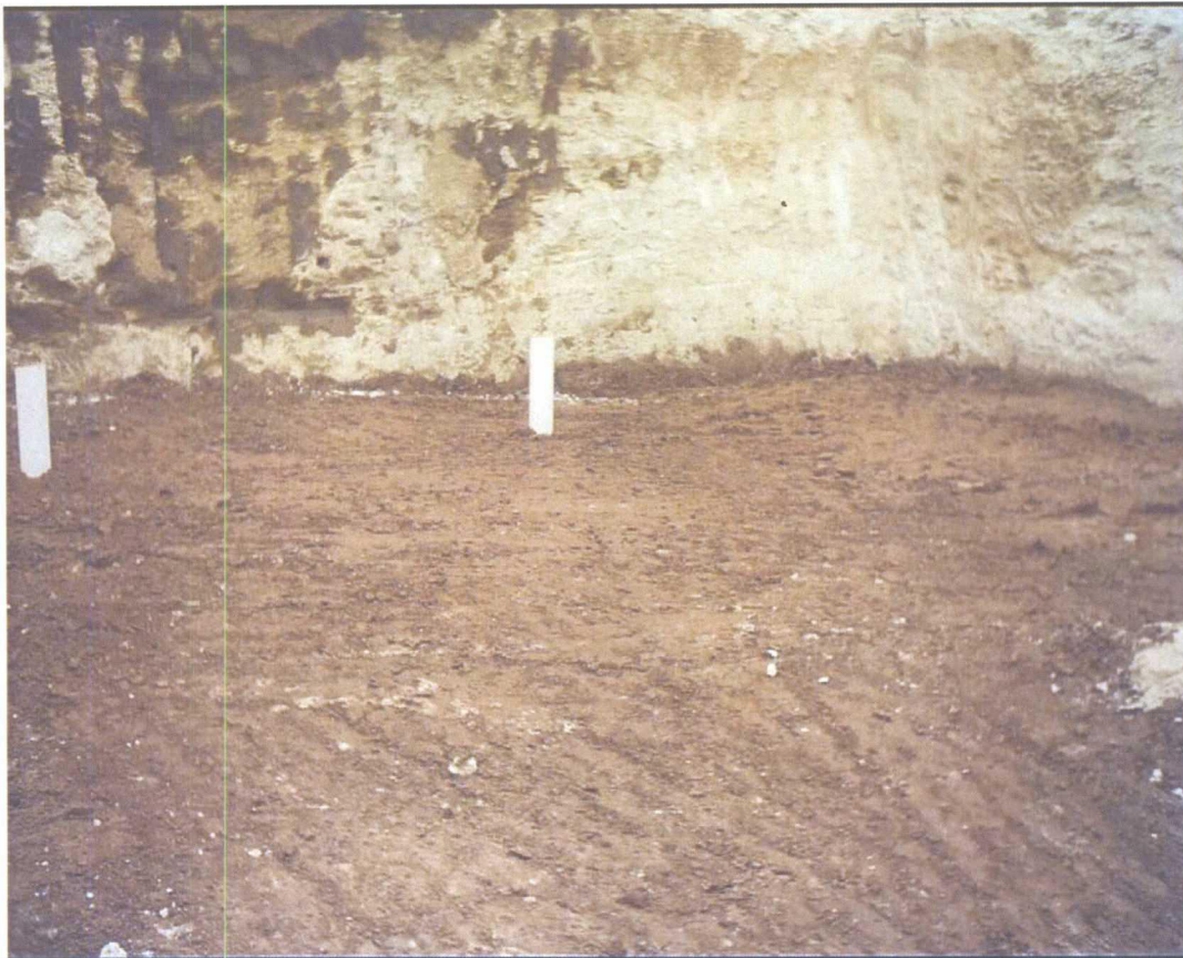
Photograph 9: Additional bentonite was placed around the base of wells prior to placement of the clay liner, forming a seal between the liner and well.
