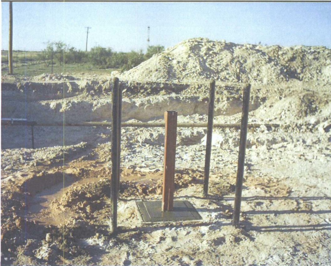
Photograph 18: A metal shroud was mounted in a two feet by two feet concrete pad adjacent to the well.
