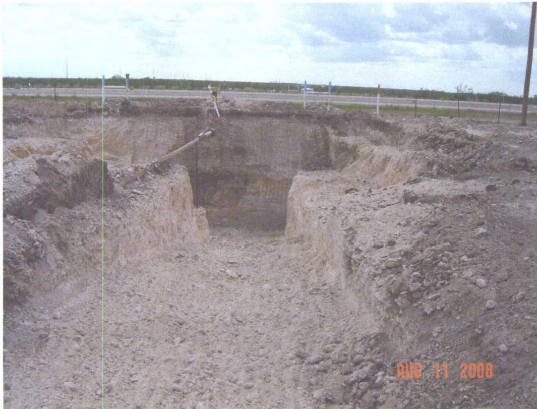
Photograph 7: The ramp into the excavation was graded with a slope of 4:1 to allow a truck mounted drilling rig access into the base of the excavation to install the passive soil vapor ventilation wells and 4 soil borings.
