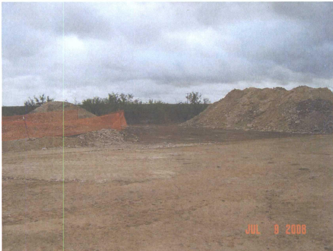
Photograph 2: A view of the north side of the excavated area where clean soil was removed and stockpiled to create ramps into the excavation.
