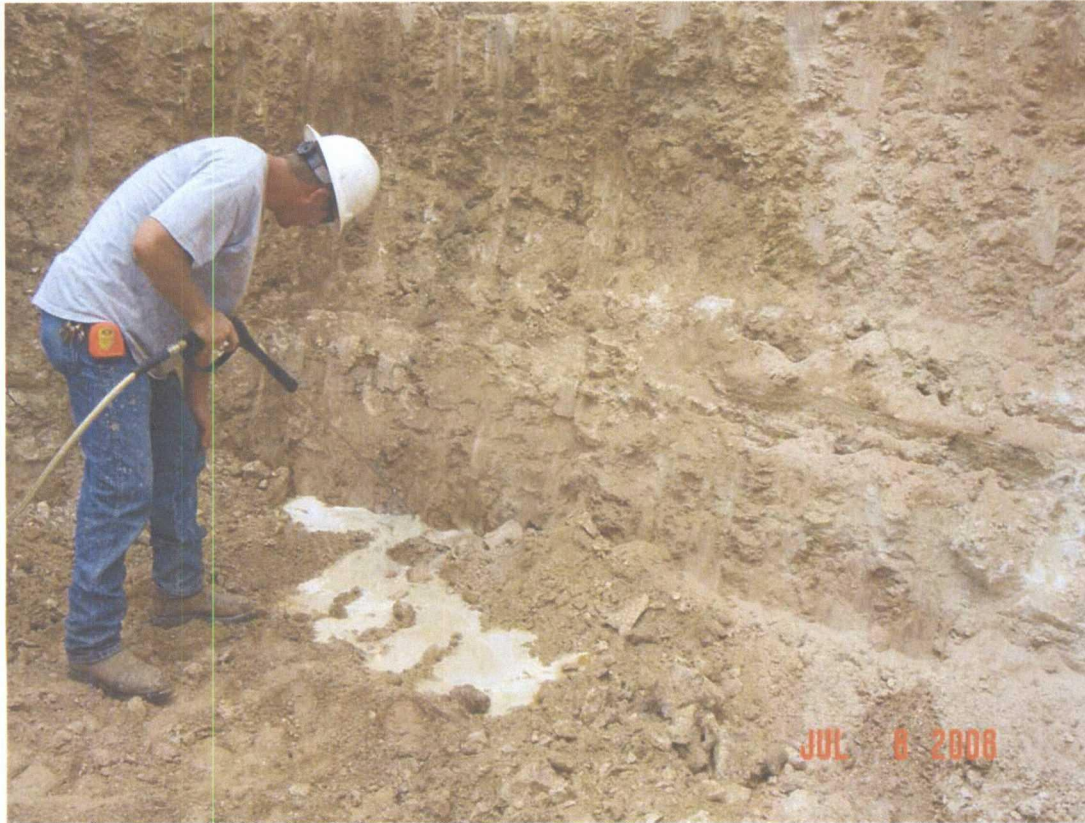
Photograph 3: A view of the west wall of the excavation, which is being treated by injecting Micro-Blaze solution.
