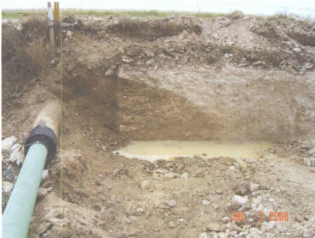
Photograph 4: A view of the west wall of the (five foot depth) excavation, treated by injecting Micro-Blaze solution.
