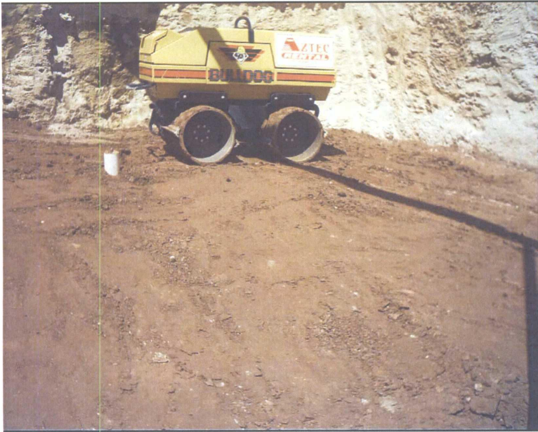
Photograph 13: The clay barrier extended at least 5-feet horizontally beyond the impacted soil in the floor of the excavation and was contoured to shed water
