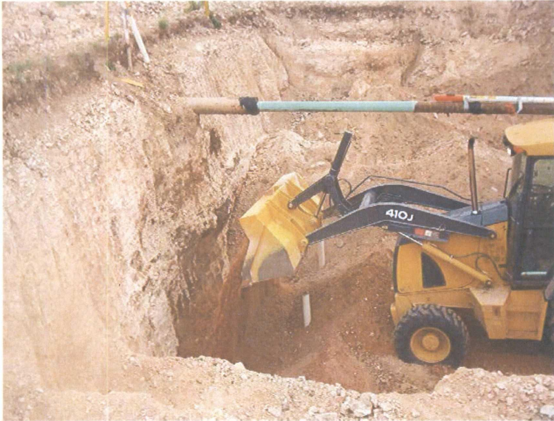
Photograph 15: Using the loader, the backfill material was placed.
