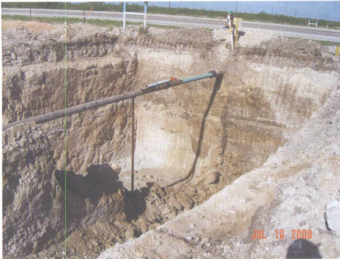
Photograph 5: Affected soils were removed until the excavation extended 22 feet from the west wall, 28 feet wide (north to south) and 19 feet deep.
