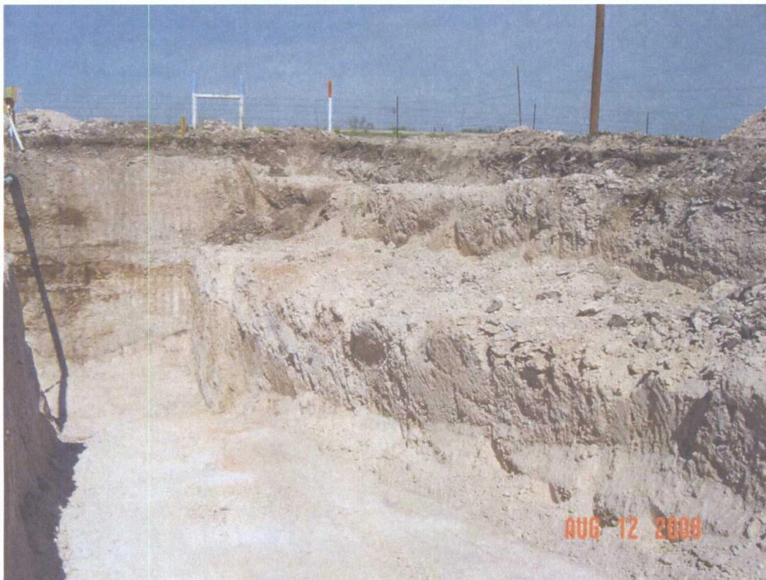
Photograph 8: The excavation was benched, prior to the installation of soil borings in the base of the excavation.
