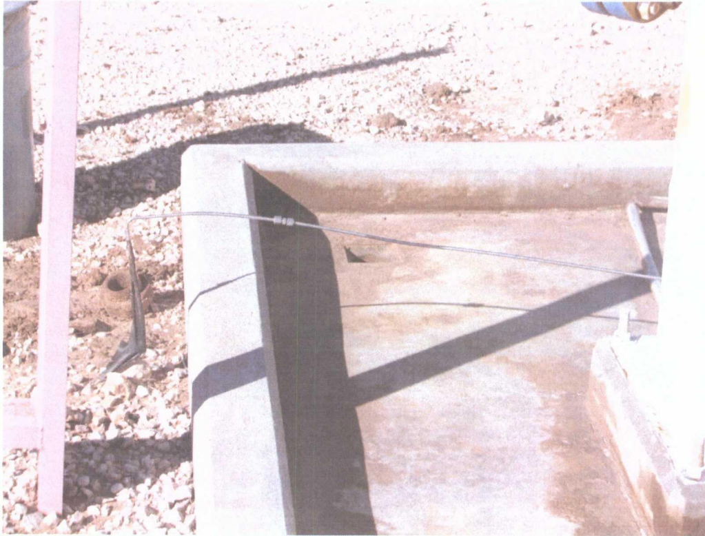
Scrubber Catch Basin with common drain opening
