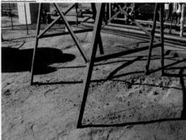
Photo 2: No secondary for saddle tank.
