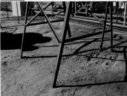
Photo 2: No secondary for saddle tank.
