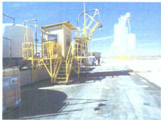
New coating on chemical concrete pad
