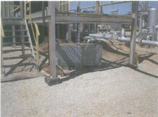
Pic#9 Electric Compressor Bldg. Sump. Single wall.
