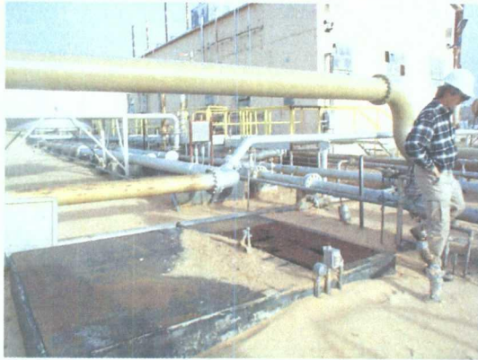
Old below grade sump collection system located west of Old Clark Compressor building.
