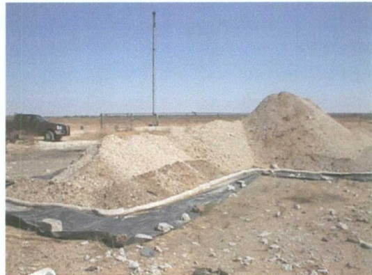
Pic#11 South plant storage area. Contaminated soil from skimmer pit remediation project.
