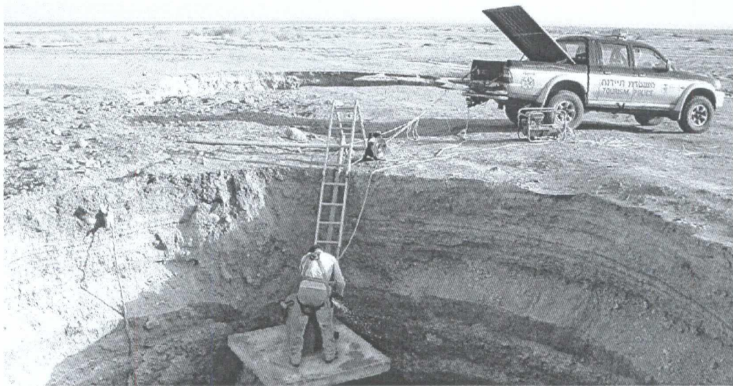
Figure 9.8. A man standing on the collar of a borehole that had dropped into a sinkhole over salt in the Israeli desert near the Dead Sea; though dissolution, cave development and sinkhole formation were already active in the area, the location of this sinkhole was determined by the borehole that was drilled to investigate the subsidence problem.
