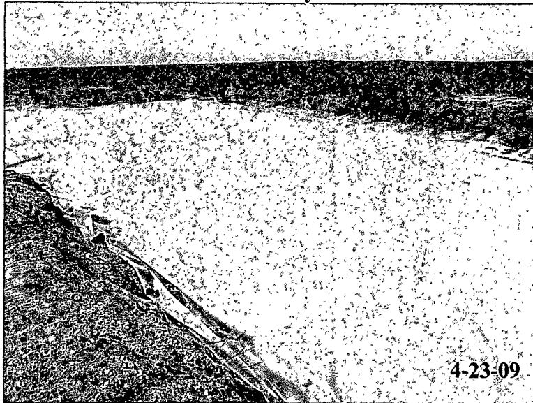
Installation of 20 mil poly liner.
