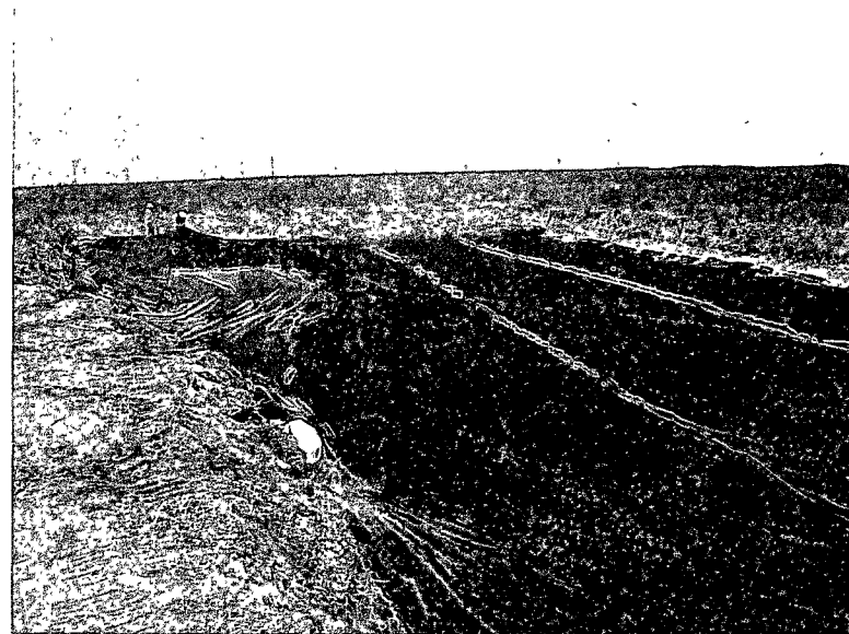
Installation of 2 nd Geotextile liner above the poly liner.
