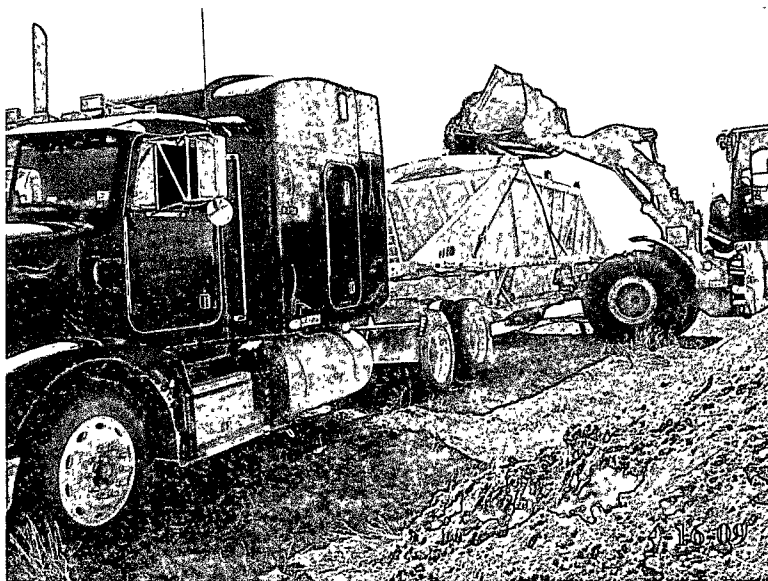
Loading impacted soil to be hauled to disposal.
