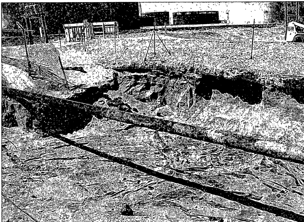
Liner installation at the Tank 374 10" Sweet Truck Haul Line (SRS 2005-00172) release
