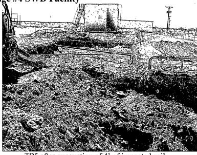
TP5 after excavation of 4' of impacted soil.
