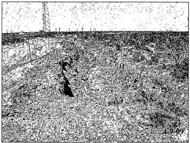
TP6, TP7, TP8 and TP9 after excavation of 4' of impacted soil.
