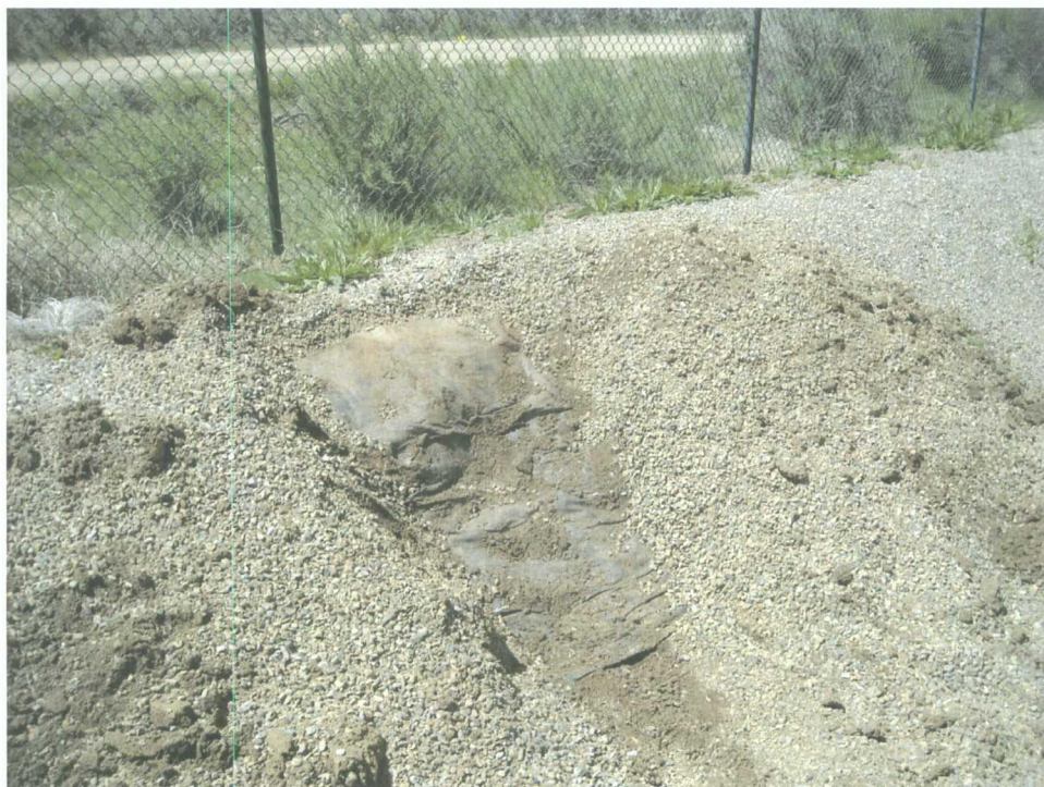
Liner under West Berm (Secondary Containment for Produced Water Tanks) (Taken May 6, 2009)
