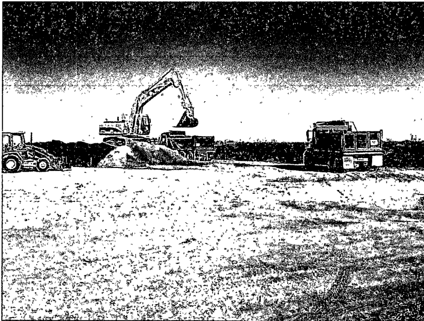
< 3/31/08 – Hauling stockpiled contaminated soil to landfarm
