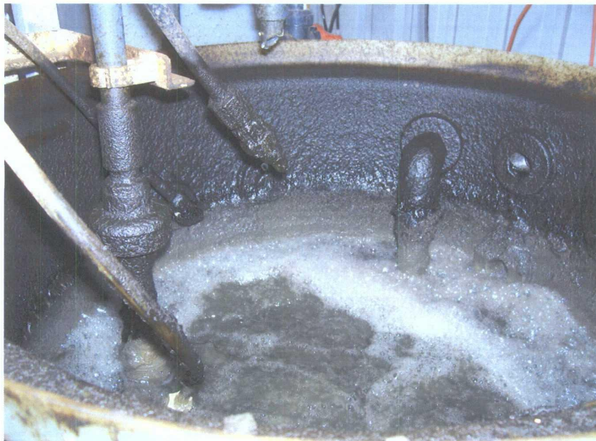
Figure D.3: Photograph of the Aerobic Tank with Submerged Membrane Filters (lower left of picture)
