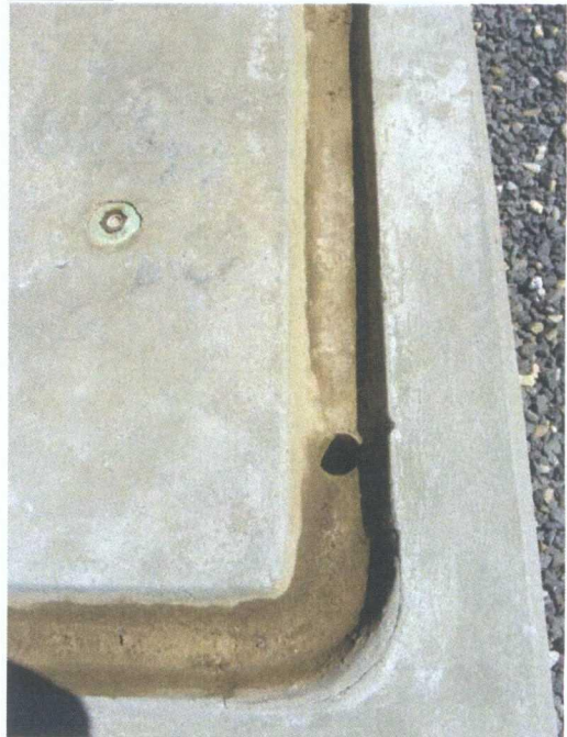
Photo 5: Unused skid with open drain.
