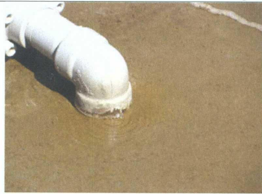
Photo 4: Gas leak within containment.
