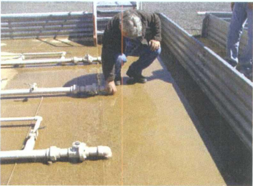
Photo 3: Verifying bubbles of conduit.
