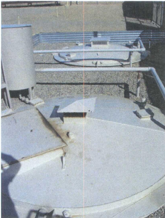
Photo 1: Two 70 BBL below-grade tanks.
