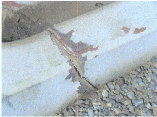
Photo 6: Cracked noted in skid.
