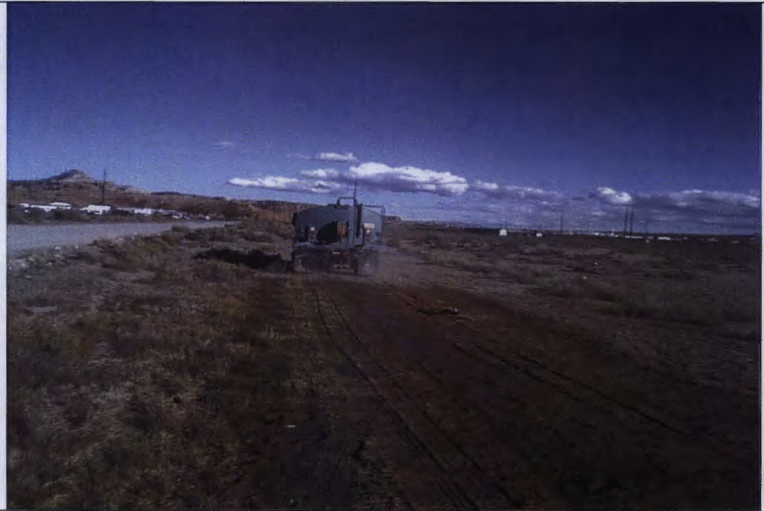
Photo No: 1 – RAD#14-0109 - EPNG Line No. 1301 Pipe Replacement Project Location: Section 8, Township 15 North, Range 17 West, McKinley County, New Mexico Comments: Photo of discharge water being used for dust control on the ROW.
