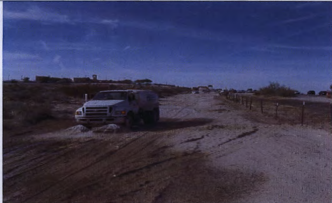
Photo No: 2 – RAD#13-0050 - EPNG Line No. 1004 Relocation Project @ NM Highway 404 Location: Sections 25 & 30, Township 26 South, Range 3 and 4 East, Dona Ana County, New Mexico Comments: Photo taken of discharge water being used for dust control on the ROW.
