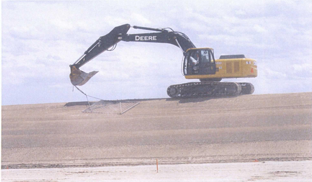
10. 6-9-09 Use of a metal grate to clear dirt clods from sideslopes
