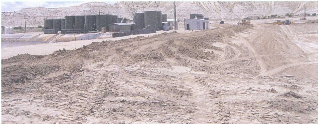
6. 6-1-09 Soil placement for additional lifts on southern berm
