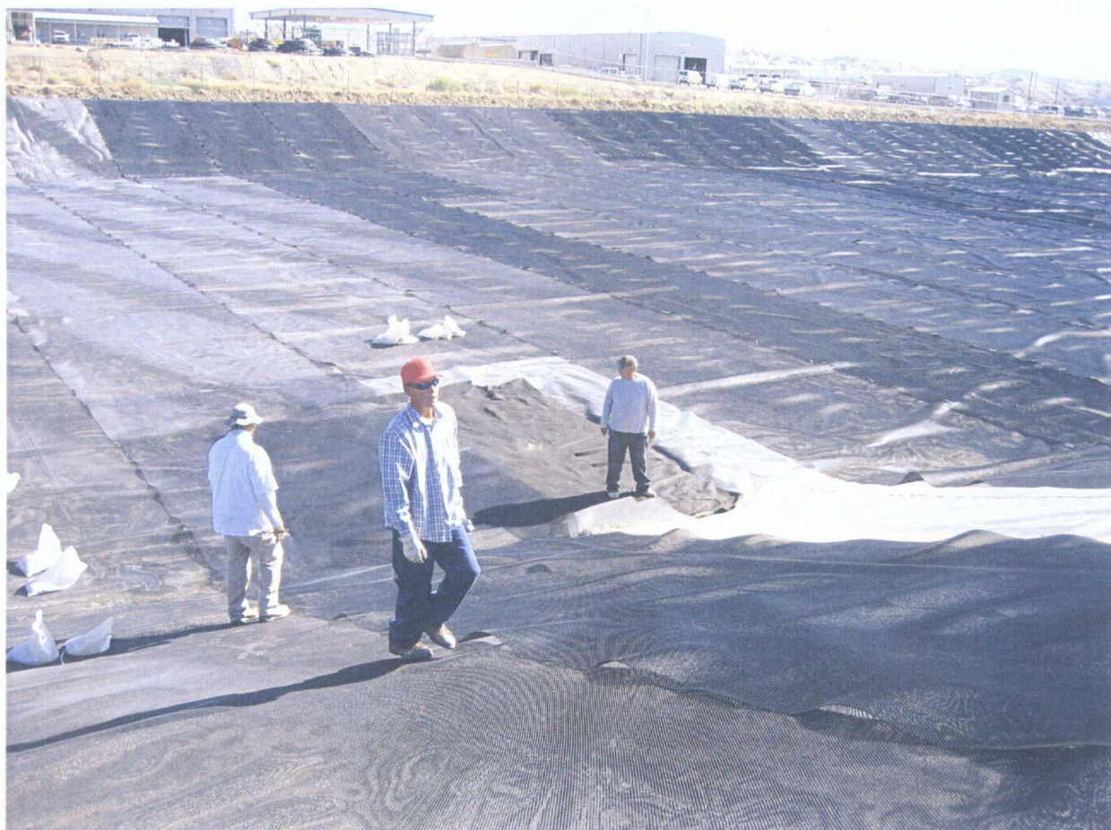
54. 6-22-09 Installation of geonet over leak detection sumps and riser pipes
