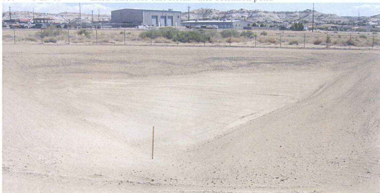
75. 6-29-09 Excavation for east stormwater detention pond
