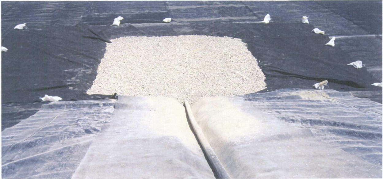
49. 6-18-09 Leak detection sump filled with aggregate
