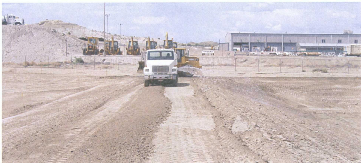
8. 6-2-09 Application of water for compaction of soils used in berm construction
