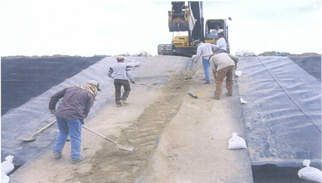
52. 6-18-09 Installation of protective soil around leak detection riser pipe
