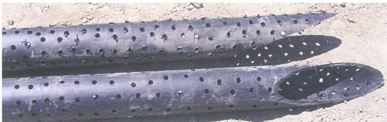
20. 6-15-09 Holes drilled in leak detection riser pipes
