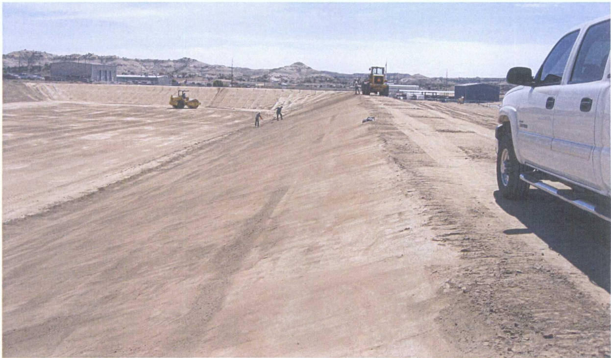
11. 6-11-09 Use of rakes, brooms and shovels to complete cleaning of sideslopes
