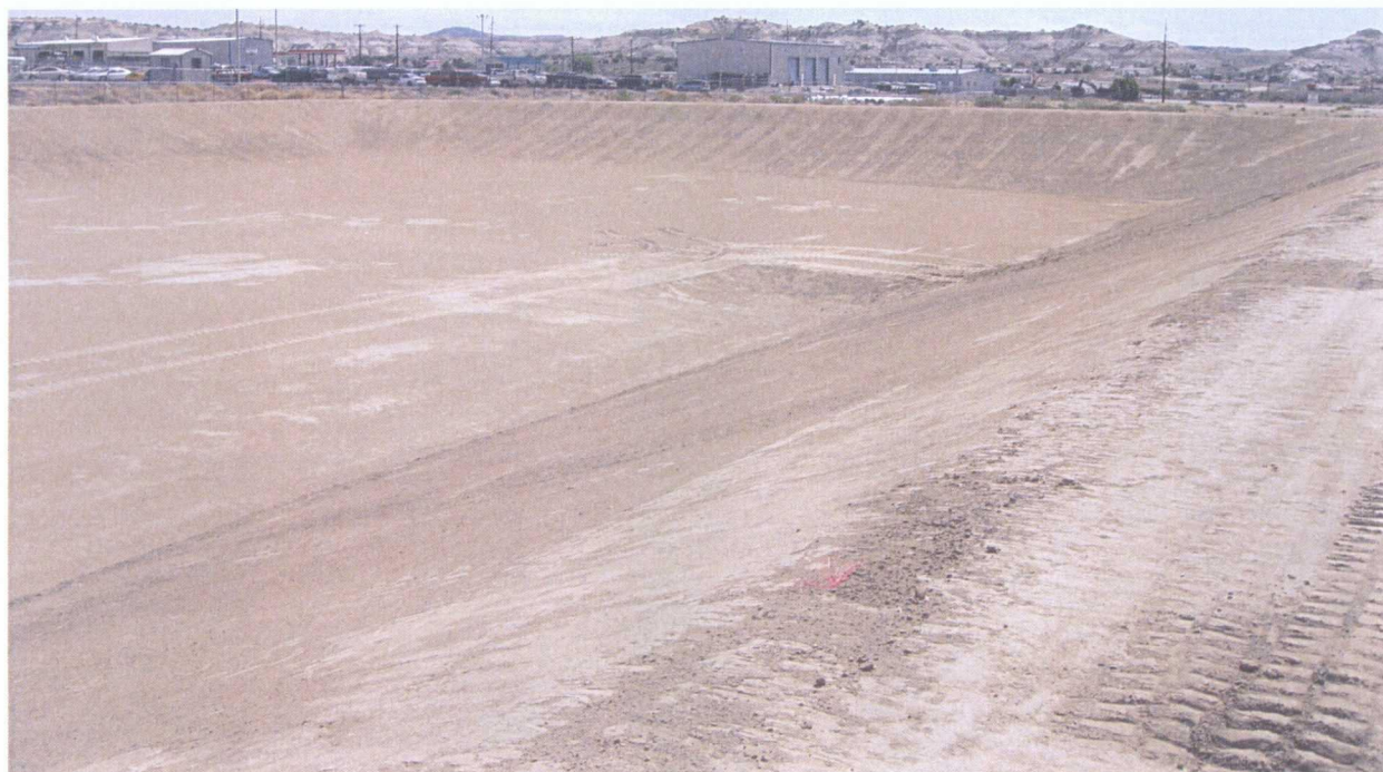
15. 6-15-09 Pond construction complete and ready for lining
