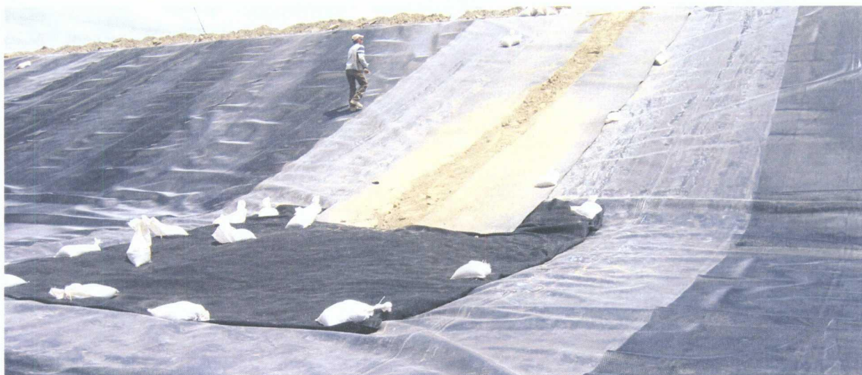
53. 6-18-09 Completed leak detection system
