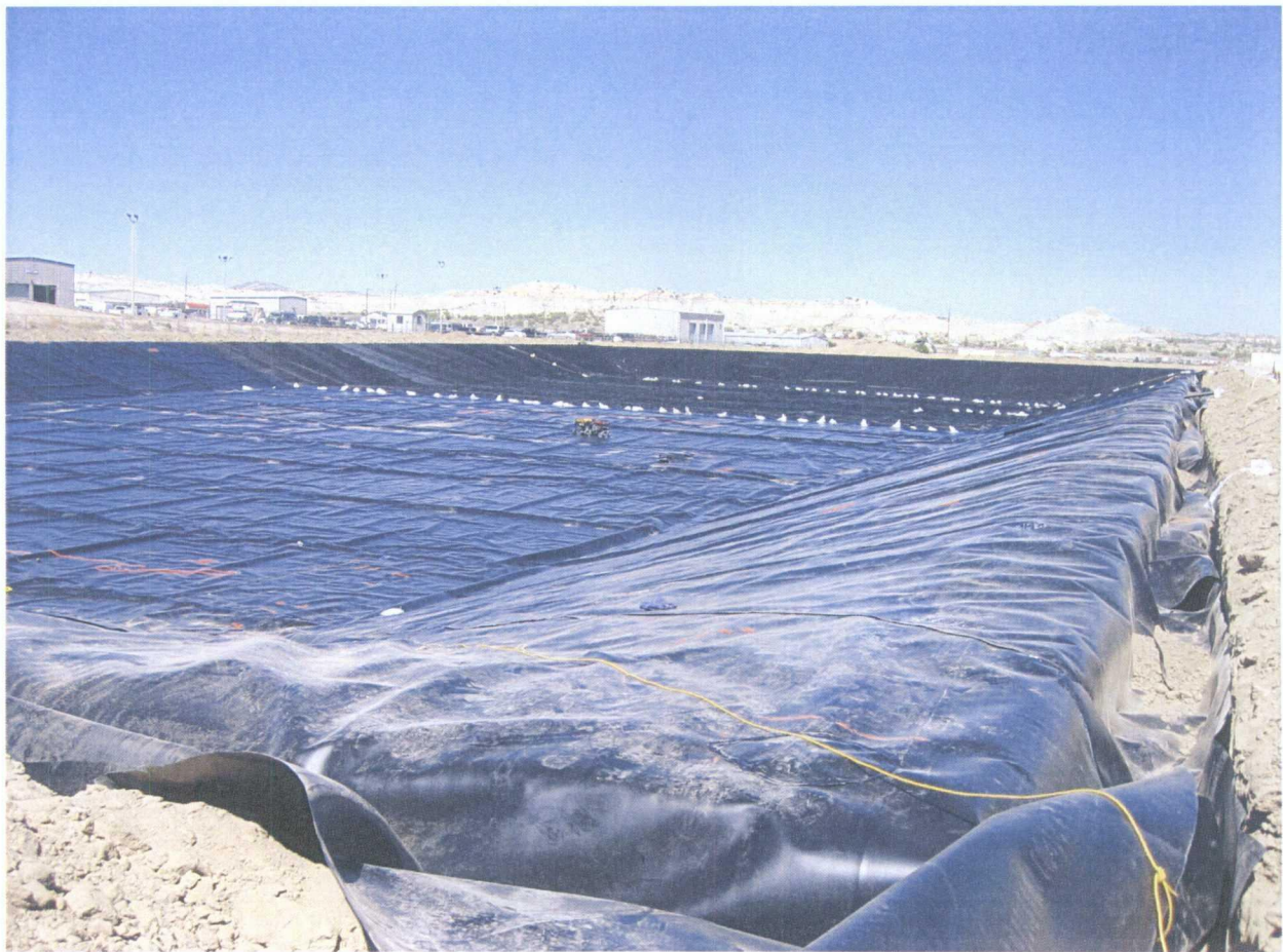
64. 6-22-09 End of day progress – Primary liner placement
