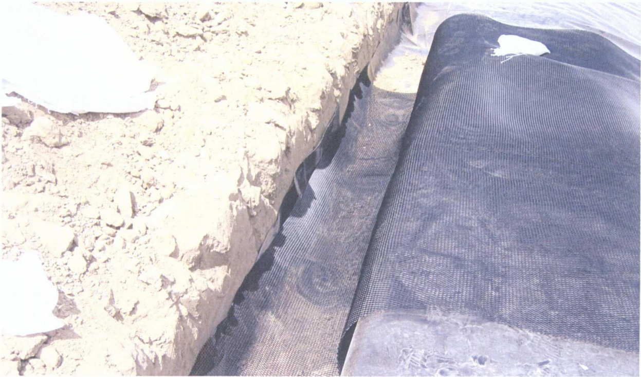
38. 6-17-09 Geonet installation in anchor trench
