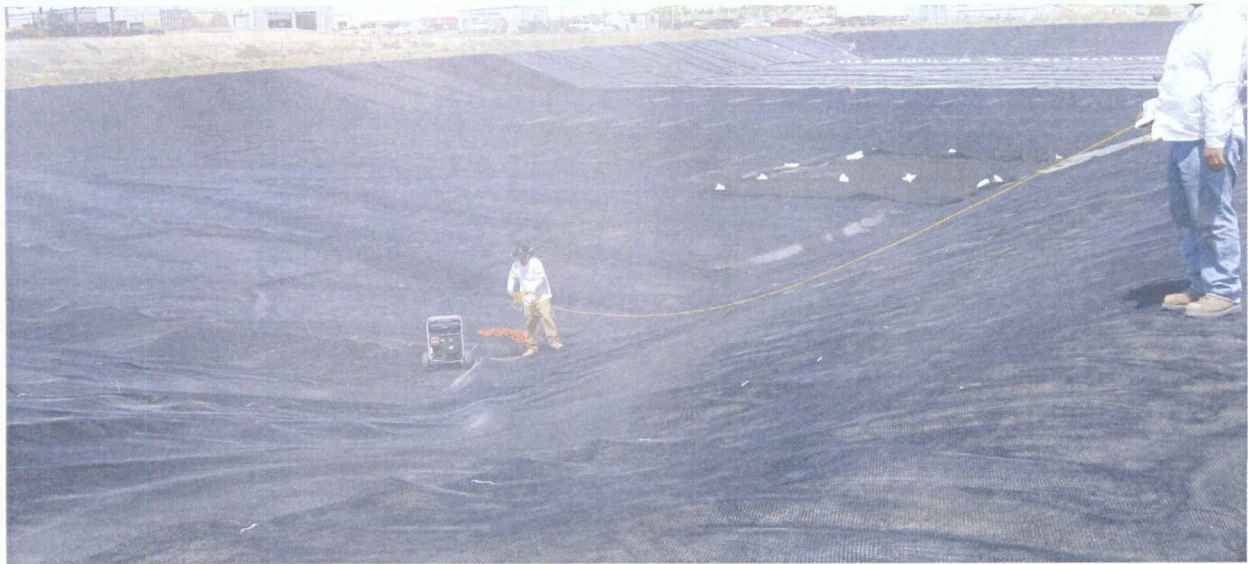
45. 6-17-09 End of day progress – Geonet placement
