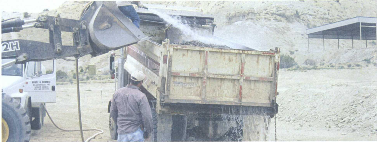
44. 6-17-09 Washing aggregate for leak detection sumps
