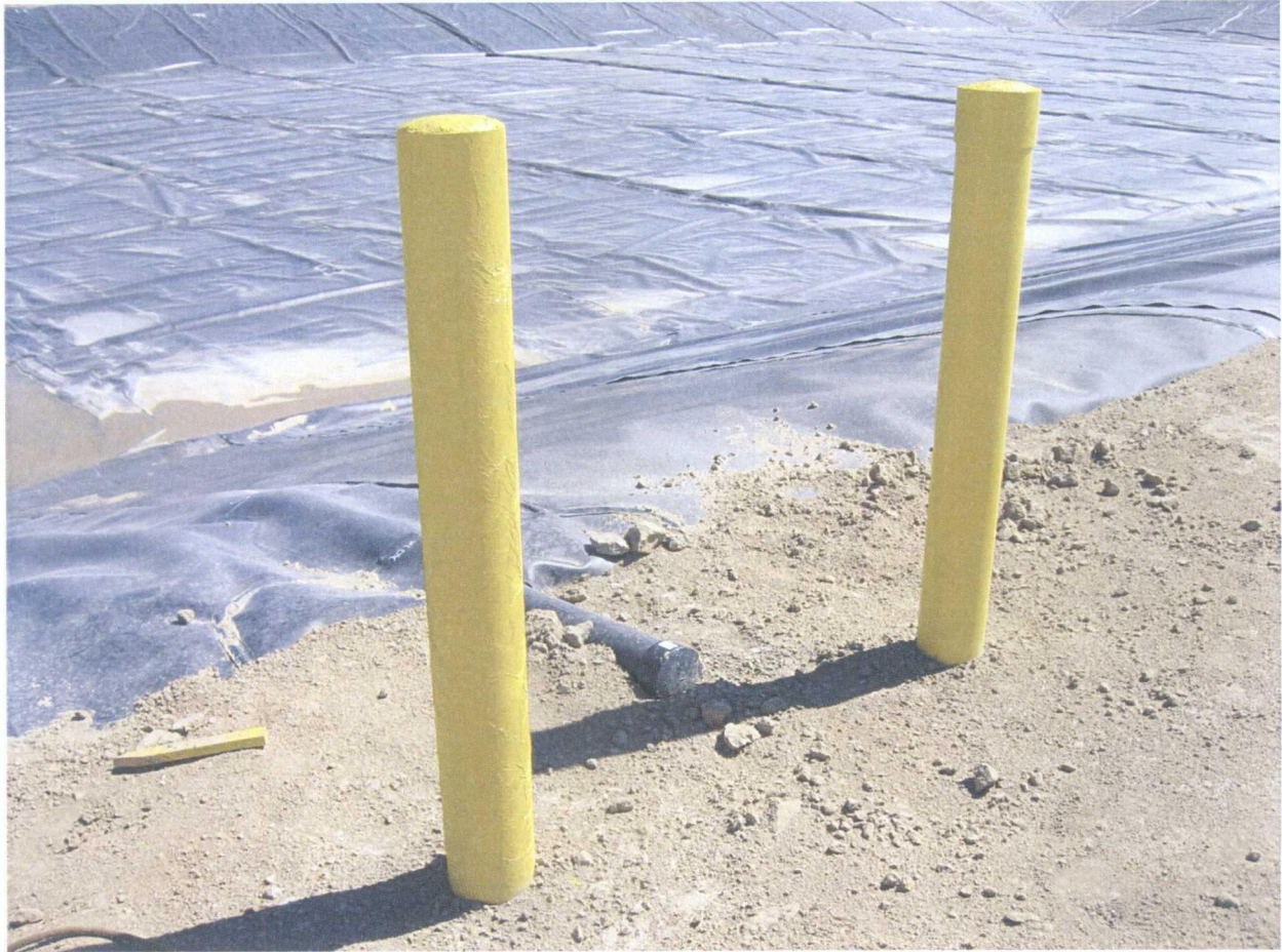
77. 7-28-09 Completed installation of Bollards protecting leak detection riser pipes.
