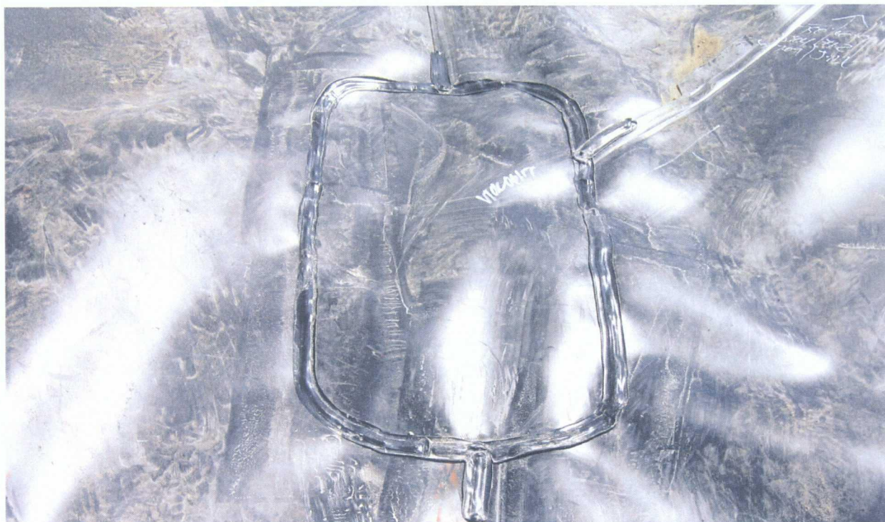
42. 6-17-09 Patch installed and vacuum tested
