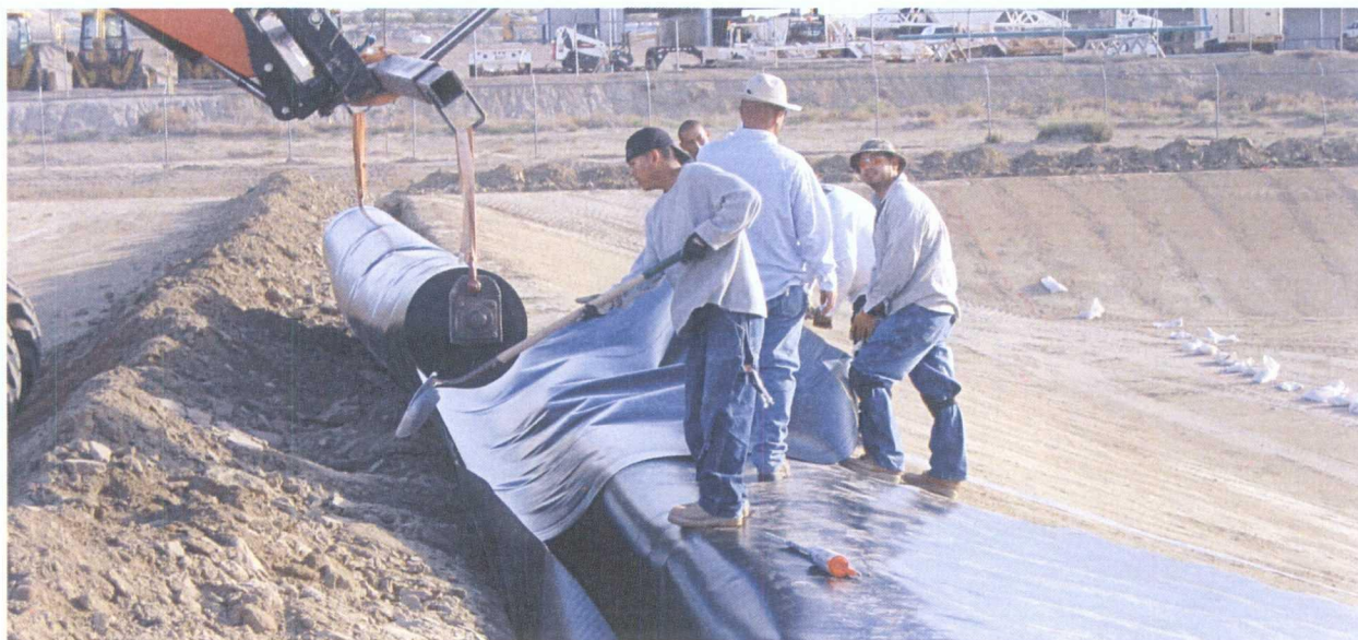
21. 6-15-09 Installation of secondary liner
