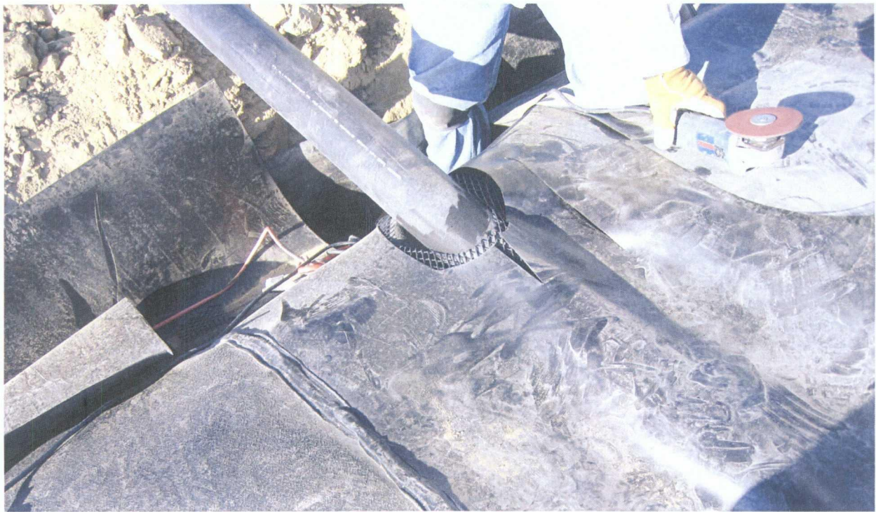
70. 6-24-09 Leak detection riser pipe extending outward from primary liner
