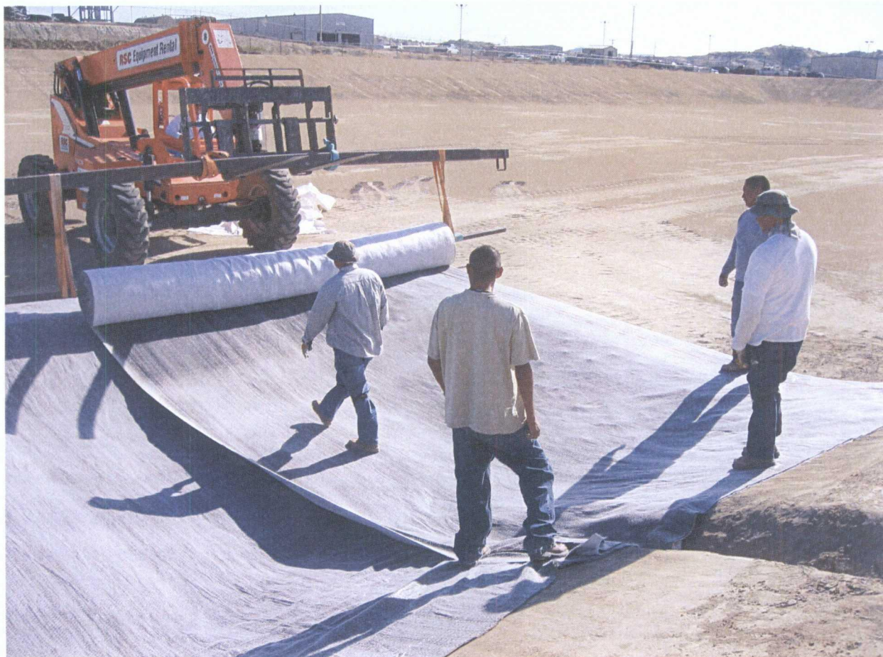
32. 6-16-09 GCL placement under leak detection sumps
