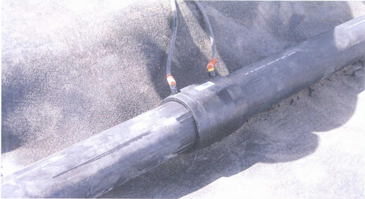
36. 6-16-09 Thermal butt fusion in progress
