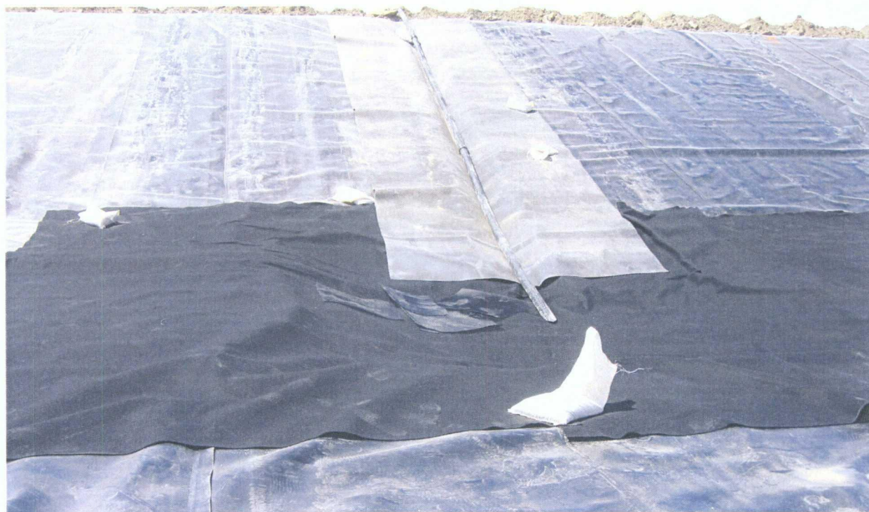
43. 6-17-09 Four geonet panels to be attached to leak detection riser pipe to protect secondary liner, and geotextile for leak detection sump construction.
