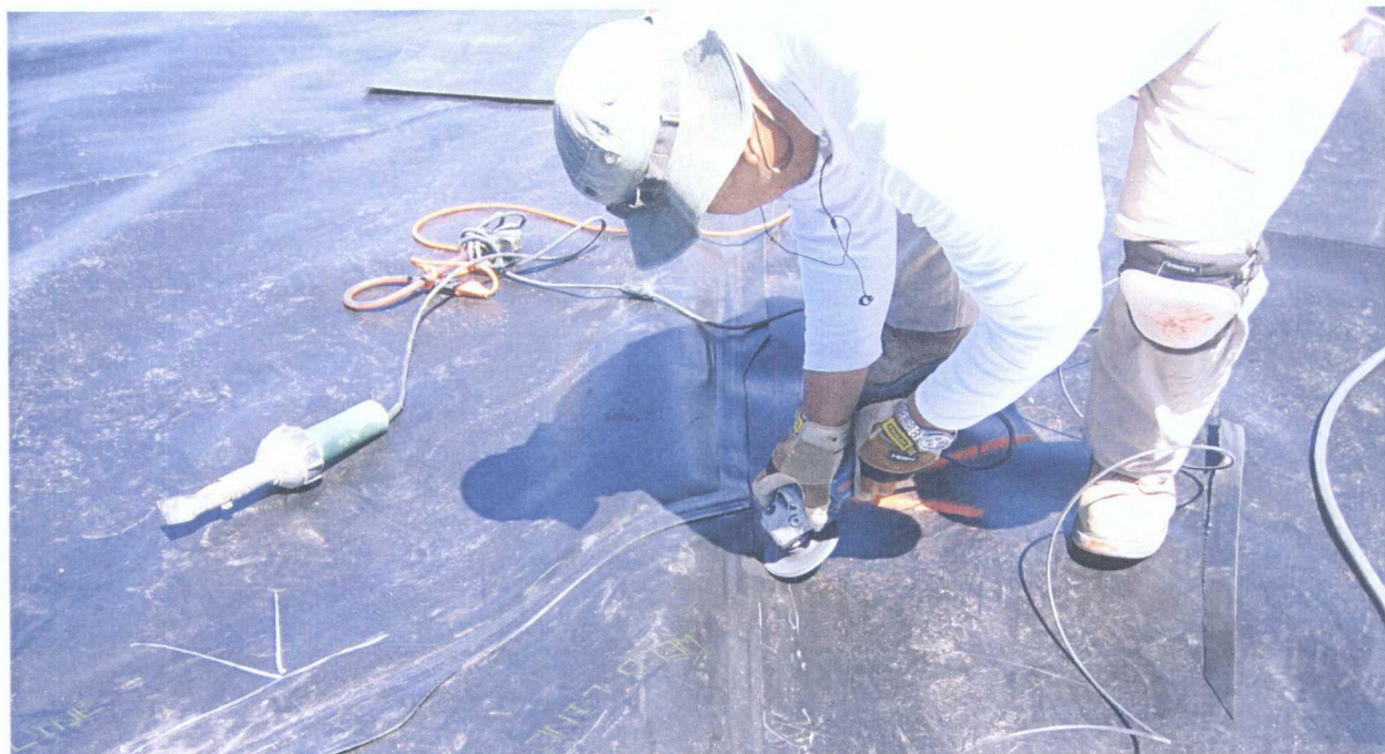
60. 6-22-09 Grinding a seam prior to extrusion welding
