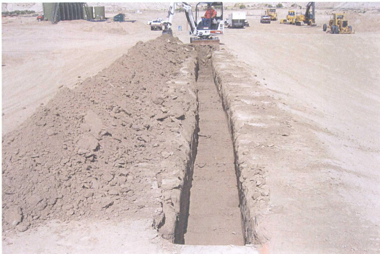
14. 6-15-09 Anchor trench construction on southern berm
