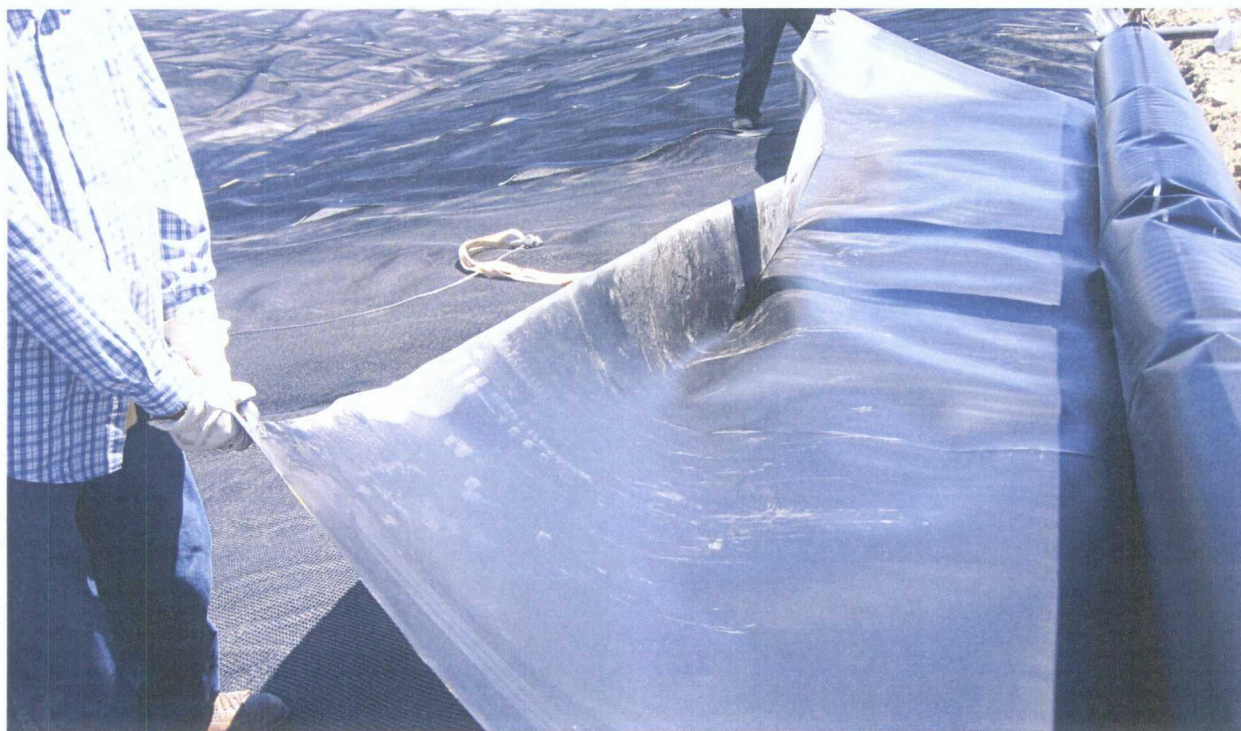
58. 6-22-09 Use of clamp and cable set up to pull primary liner across pond
