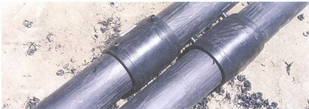
19. 6-15-09 Leak detection riser pipes fused using thermal butt joints
