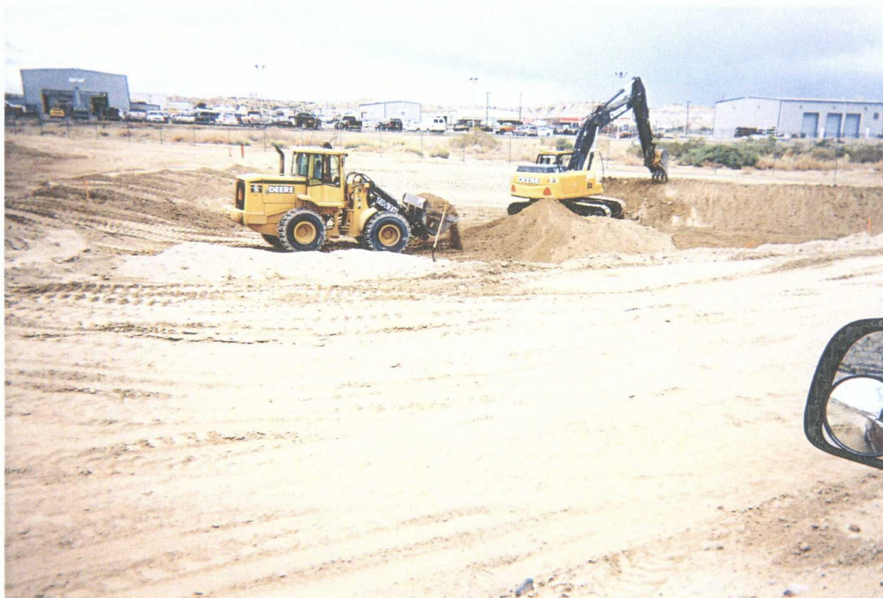
75. 6-29-09 Excavation for east stormwater detention pond
