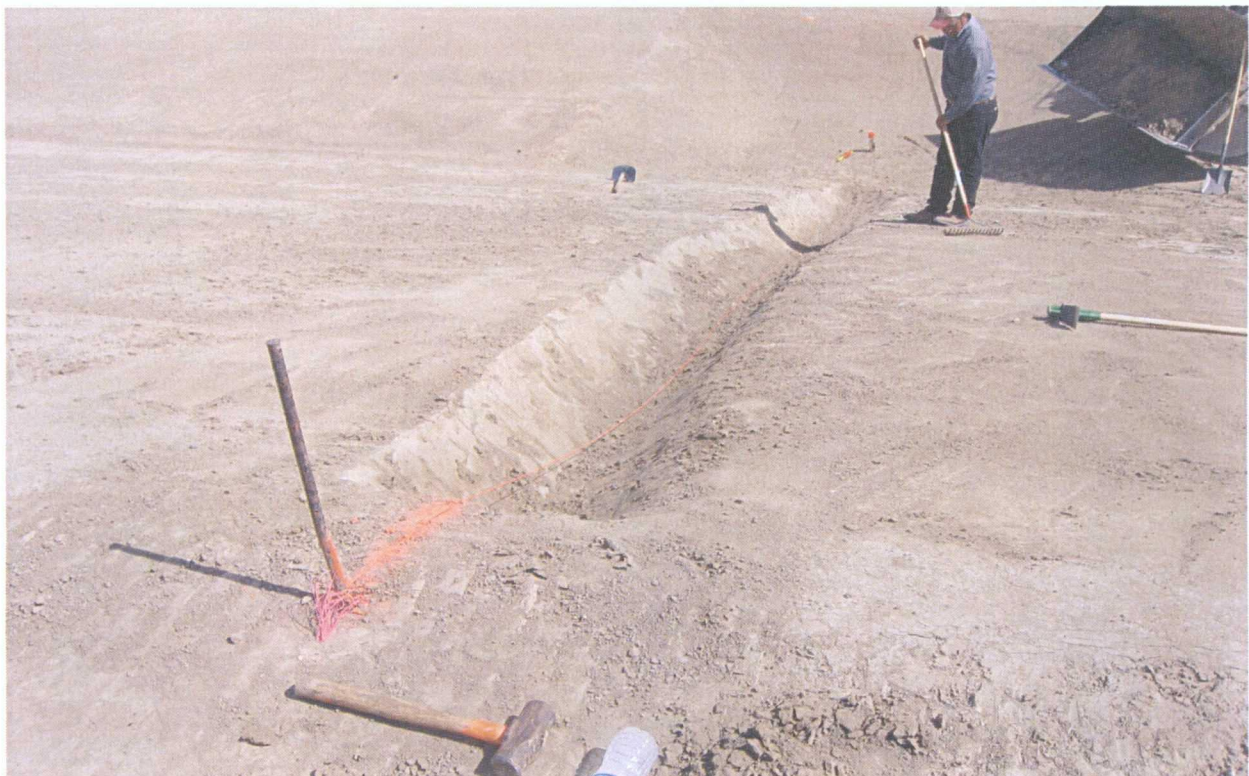
13. 6-15-09 Trench for leak detection riser pipe
