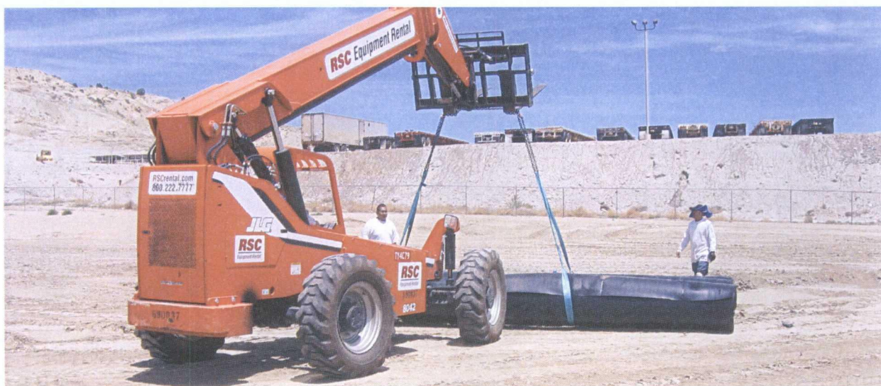
17. 6-15-09 Unloading of FML material
