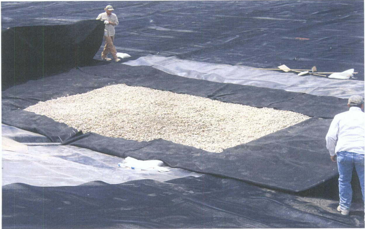
51. 6-18-09 Folding over of geotextile to “burrito” the leak detection sump
