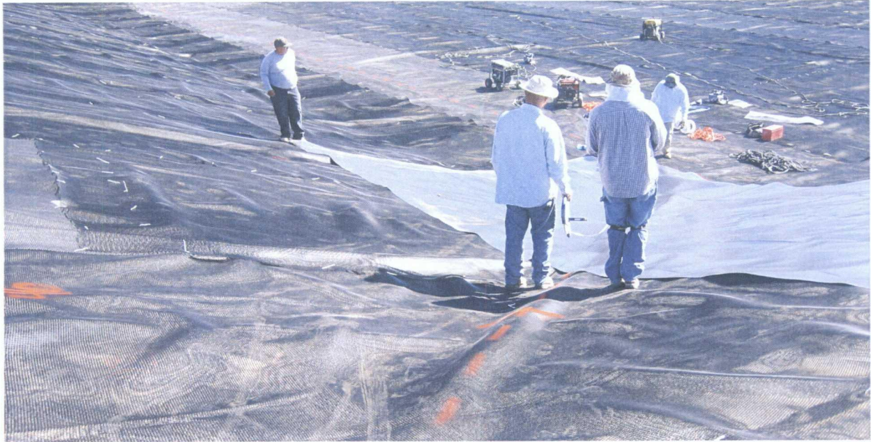
55. 6-22-09 Installation of primary liner
