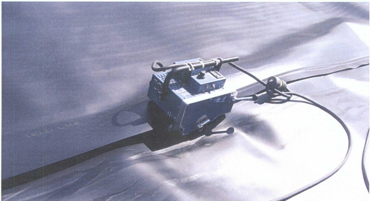
25 6-16-09 Seaming "Wedge welding" in progress
