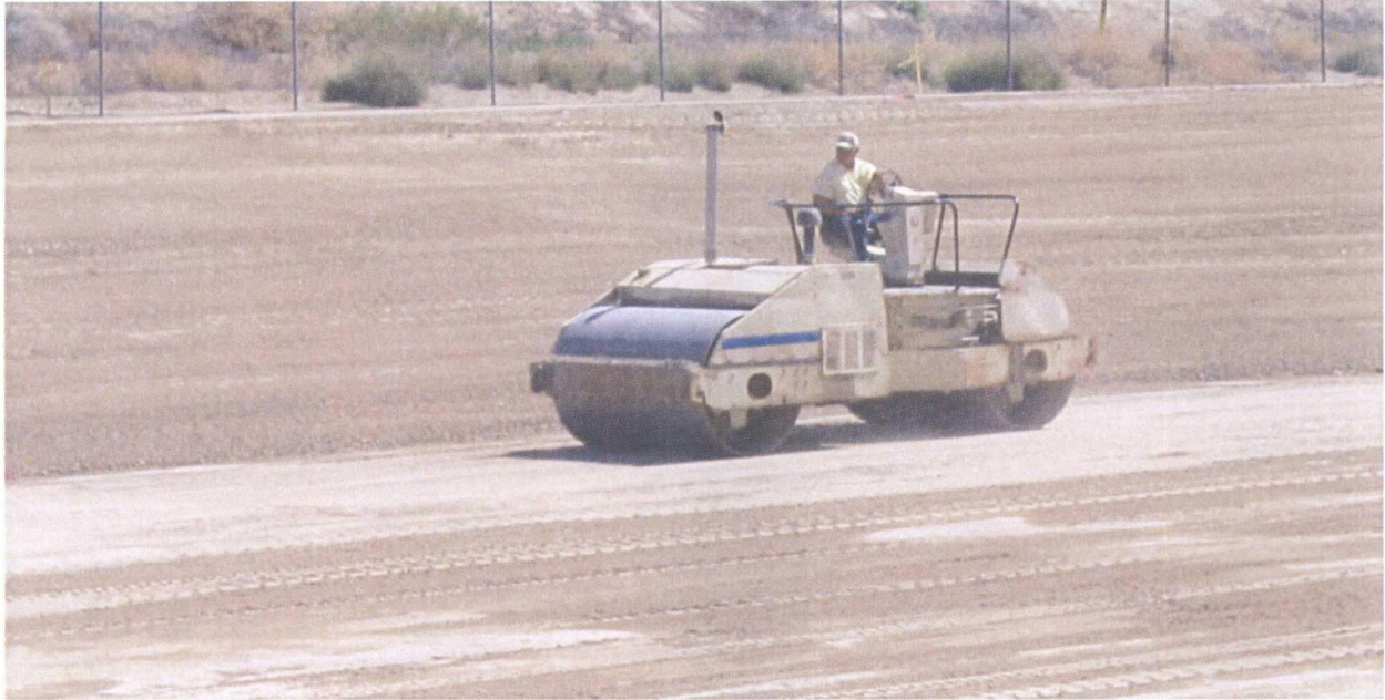
12. 6-11-09 Rolling floor of Evaporation Pond 3
