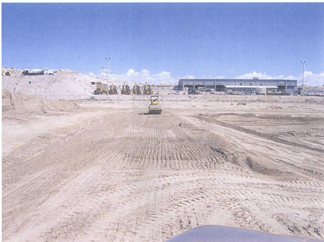
4. 5-27-09 Berm compaction during construction
