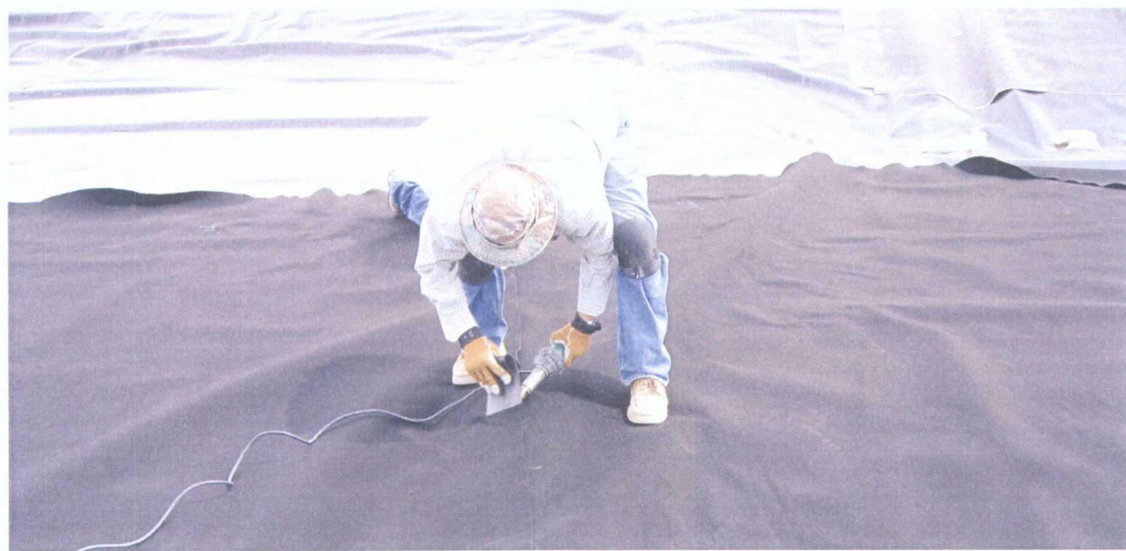
33. 6-16-09 Using Lyster to heat weld geotextile
