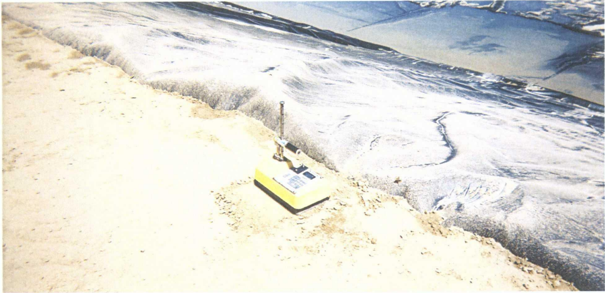
73. 6-29-09 Density testing of anchor trenches
