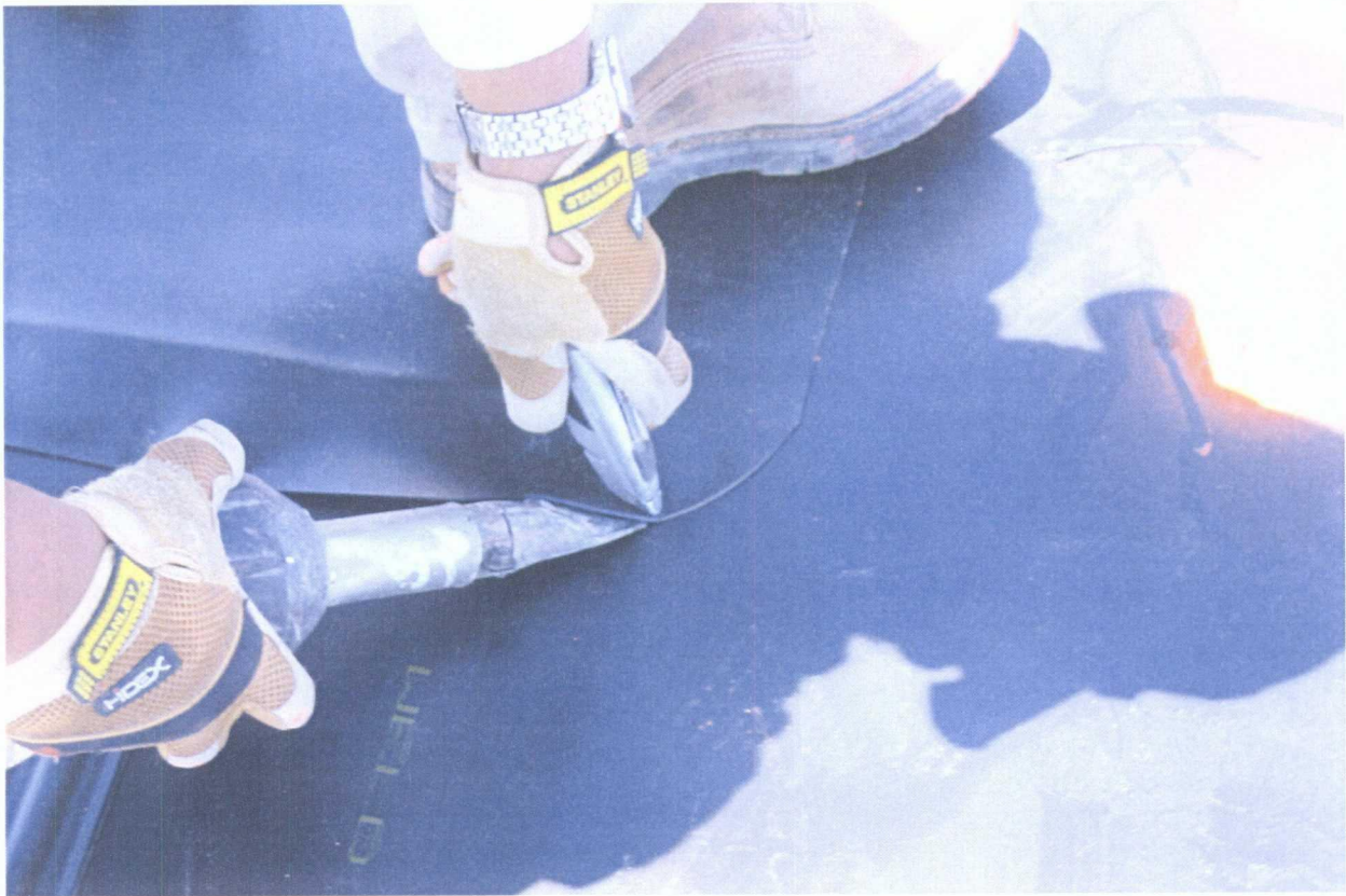
59. 6-22-09 Using Lyster to heat tack a patch prior to extrusion welding
