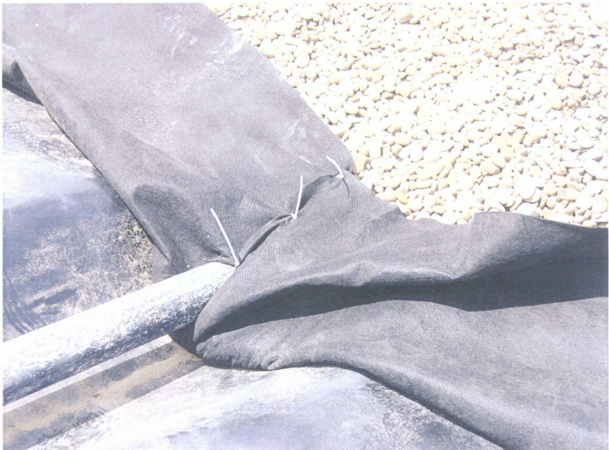
50. 6-18-09 Use of zip ties to anchor geotextile around leak detection riser pipe
