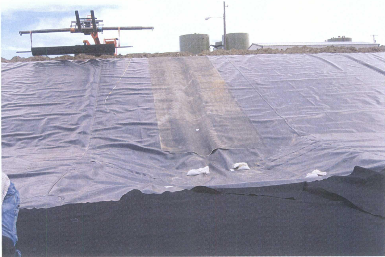
34. 6-16-09 Textured panel in leak detection riser pipe trench for soil stability
