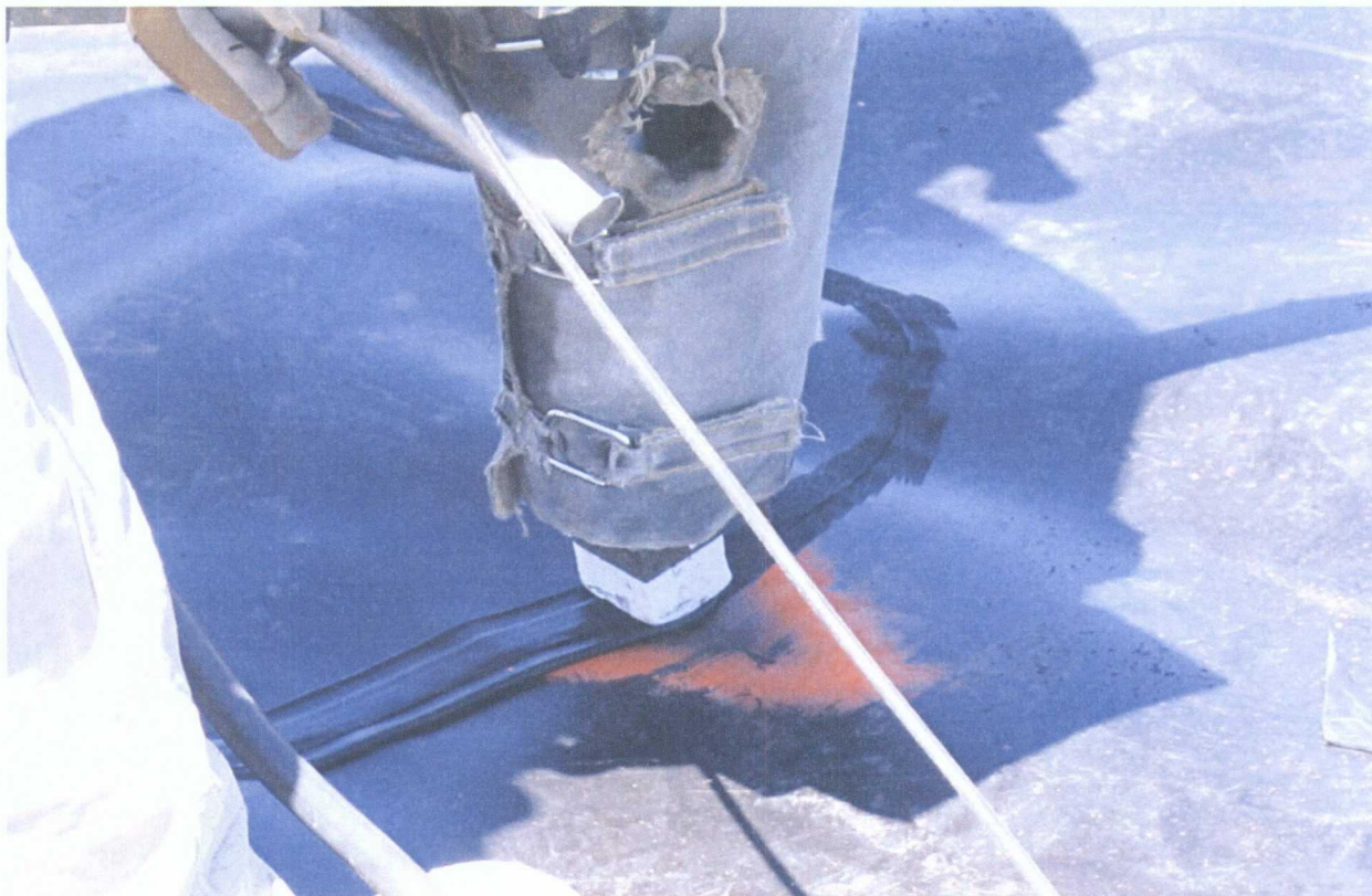
61. 6-22-09 Extrusion welding
