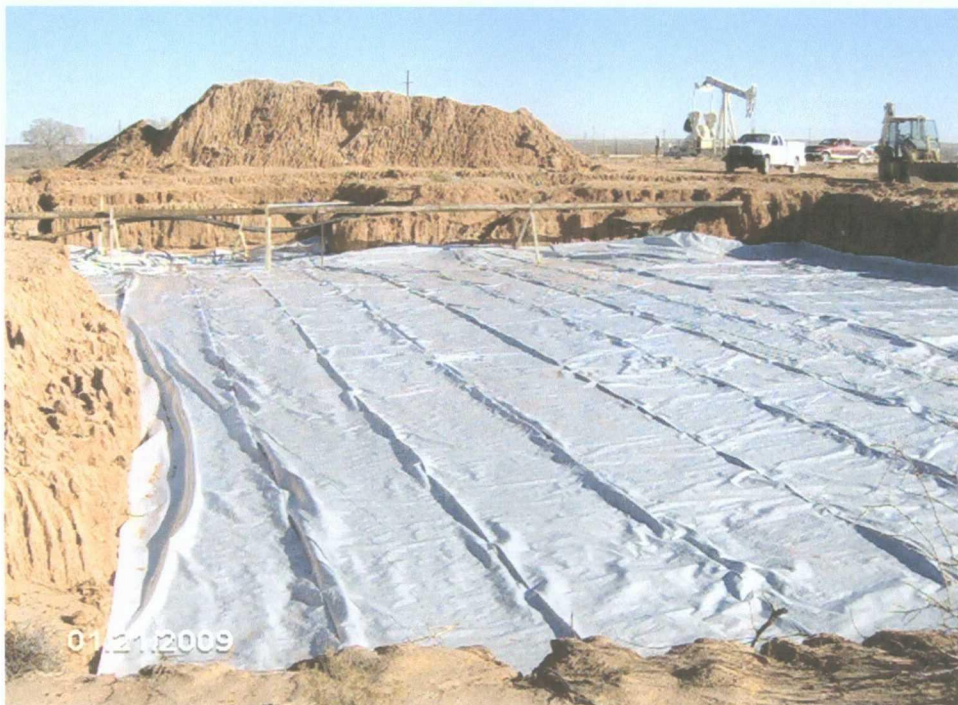
Liner Installation Looking Northeast January 21, 2009
