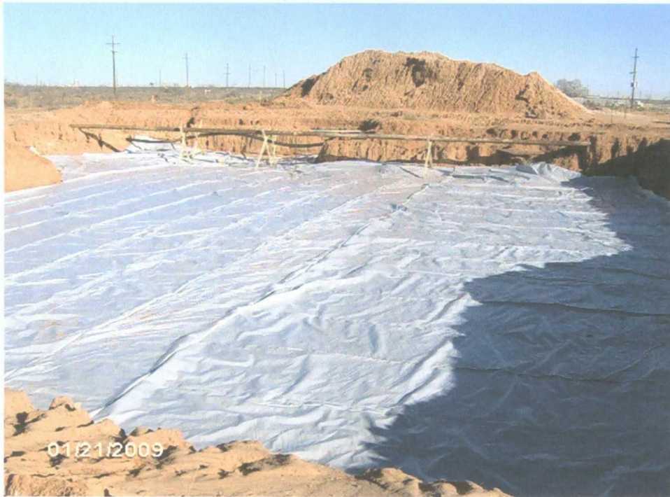
Liner Installation Looking North, January 21, 2009
