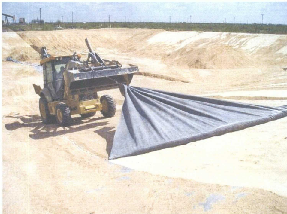
A backhoe and chain are used to remove the secondary liner. A second layer of cushion sand is between the bottom liner and native soil.
