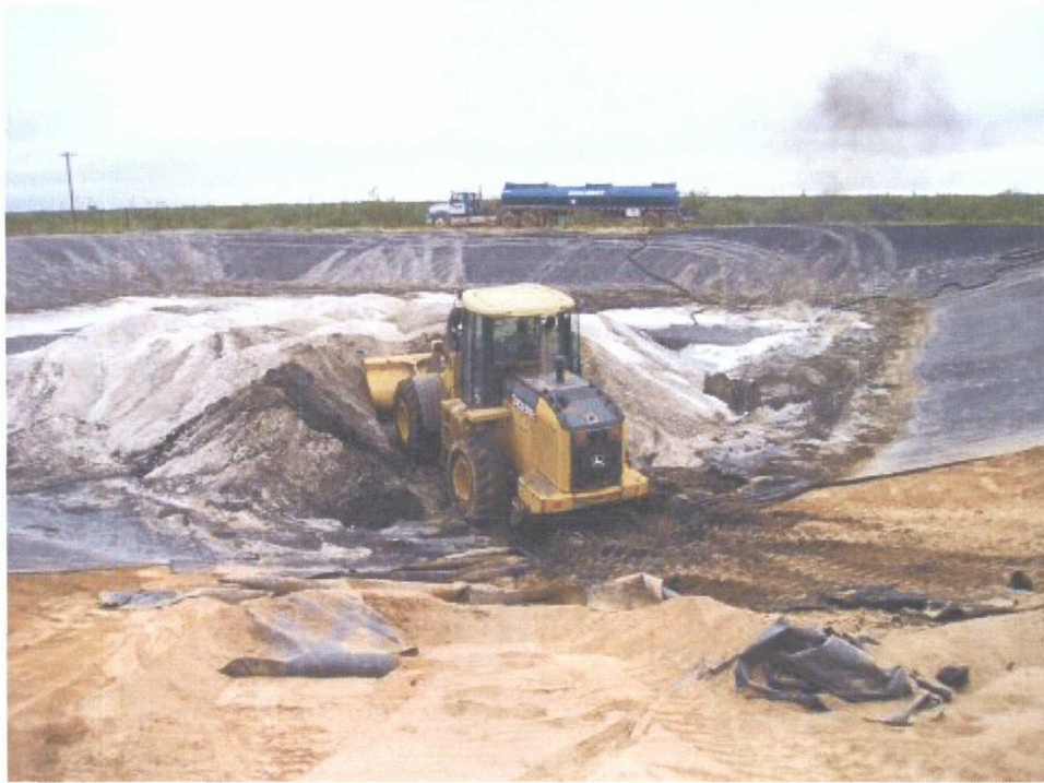
Excavated salt and sediment being stockpiled. Vacuum trucks remain onsite as liquids continue to decant from the sediment.
