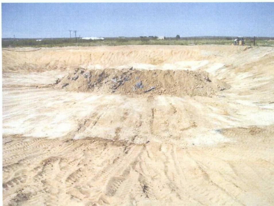
The secondary liner and cushion sand are stockpiled in the former pond pending being loaded for transport for final disposal.
