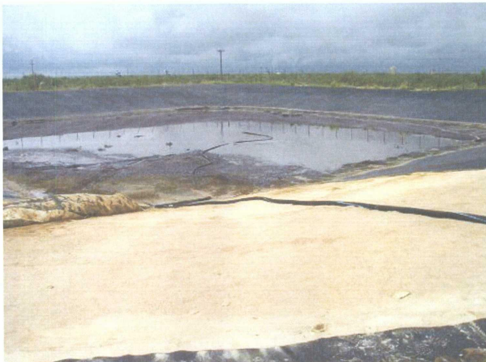
A portion of the primary (top) liner is removed to expose the intermediate cushion sand and secondary (bottom) liner.
