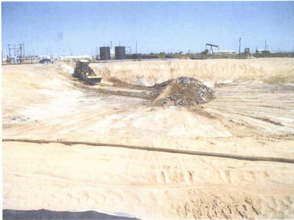
Continued progress in the upper liner removal and disposal.
