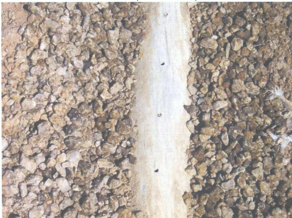
Close up of sump collection system and pea gravel filter pack.
