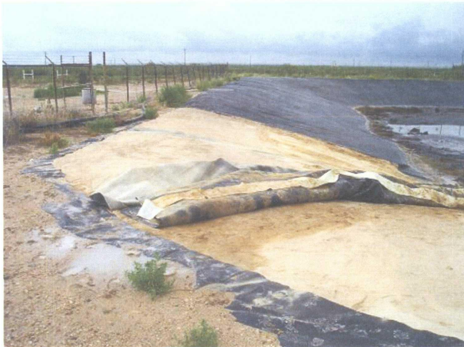
Another view of primary liner, cushion sand, and secondary liner.
