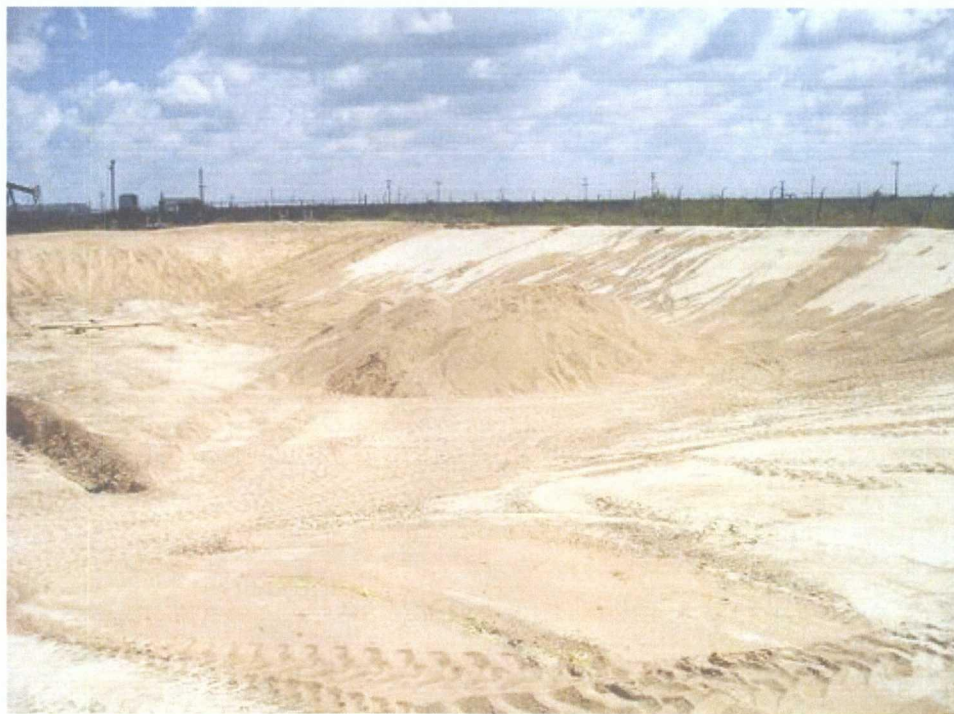
View of the former pond with both liners removed. The stock pile of sand is from layer between the secondary liner and native soil.
