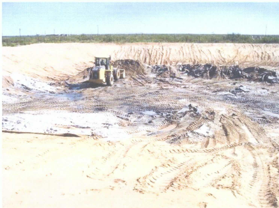
With most of the precipitated salt and sediments removed, the upper liner portion is removed from the sloped walls.
