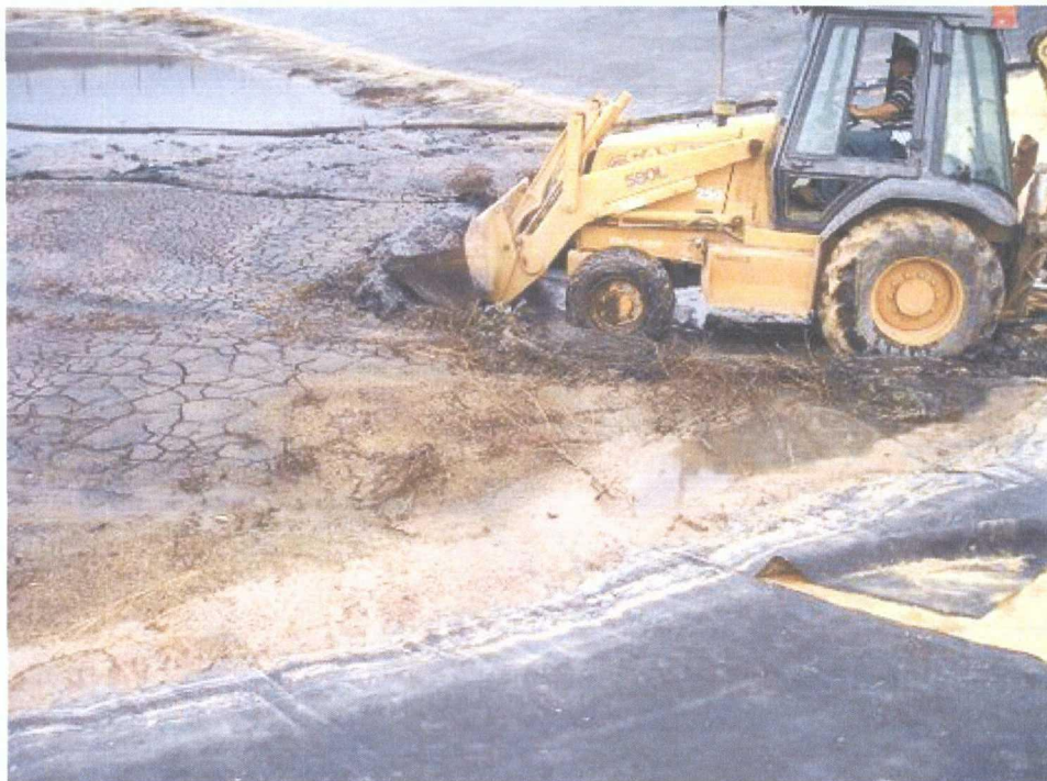
Precipitated salt and sediments are pushed towards the center to encourage decanting liquids for disposal, and to create a solid material stockpile for removal.
