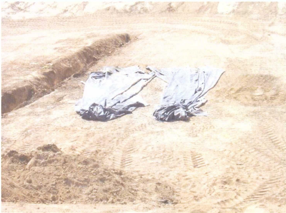
Bottom liner removed from the leachate collection system.
