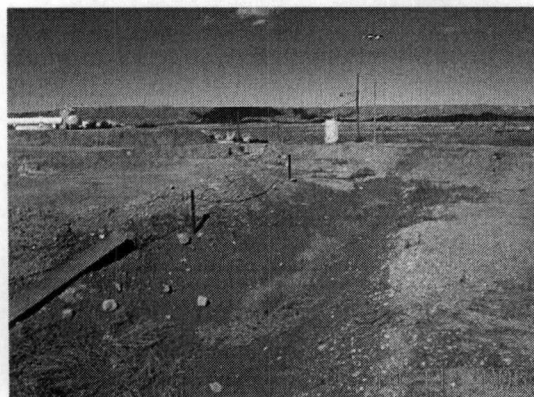
Looking northward toward NE region of process area where ponding from overflow of fire water and diluted HF acid flowed to NE corner of process area to pond within berm
