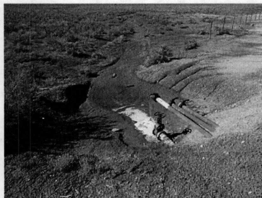
Outfall area #1 at west side of refinery. Note, outfall area #2 has been closed with a new storm water diversion setup closer to the plant. SWPPP recently completed for EPA depicts new storm water drainage diagram. Giant has not been contacted by EPA based on the submittal.
