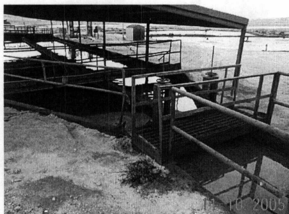
Old API separator near flare stack w/ roof needs fluid removal, used in conjunction with recently install New API separator
