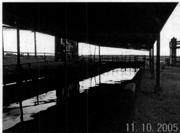
Old API separator near flare stack w/ roof needs fluid removal, used in conjunction with recently install New API separator
