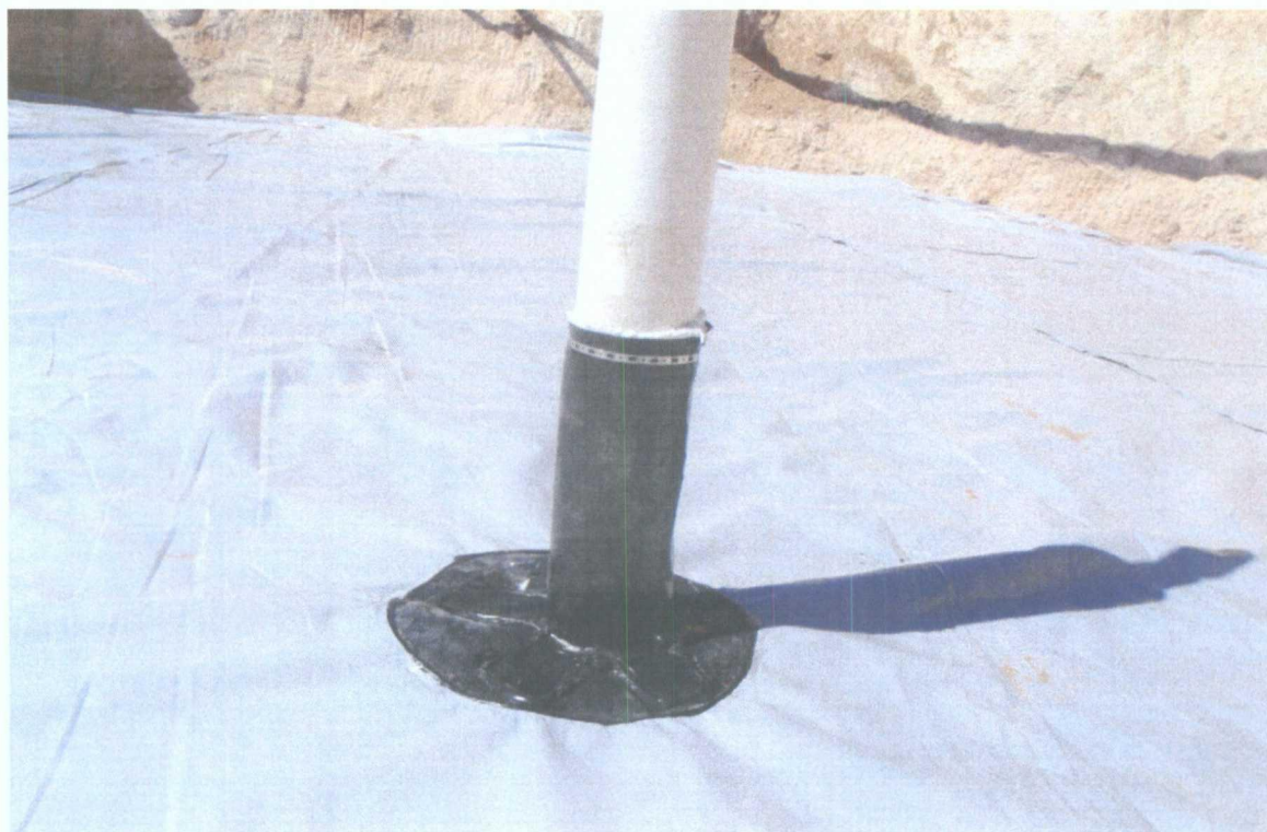
Red Byrd Ranch Historical, Chemically Welded Boot to liner
