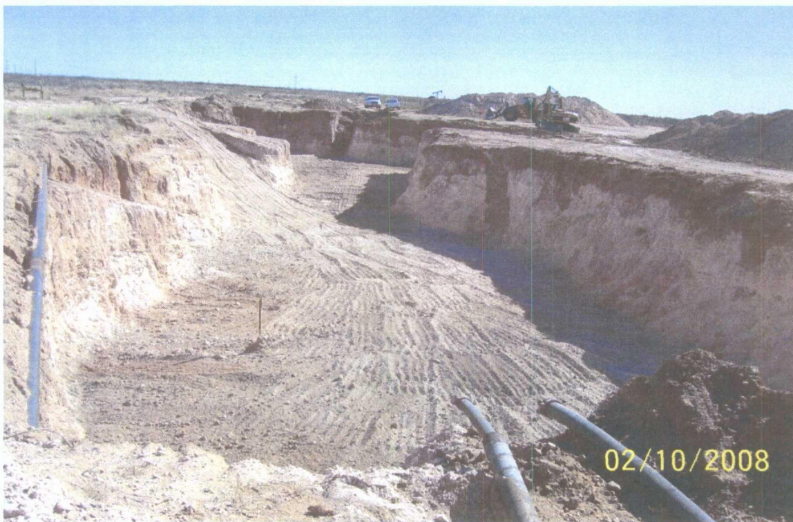
Red Byrd Ranch Historical, Excavation Completed, Pad Sand for liner placed in Excavation (Looking East)
