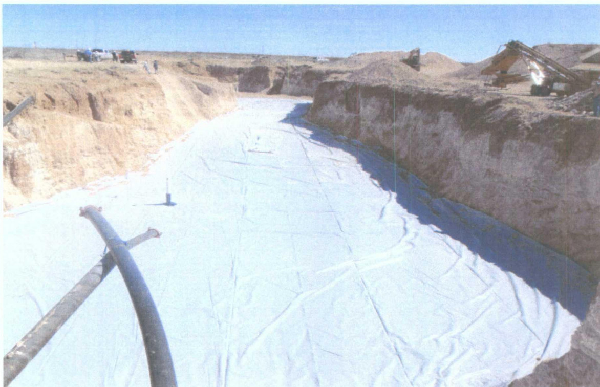
Red Byrd Ranch Historical Liner Installation Completed (Looking East)
