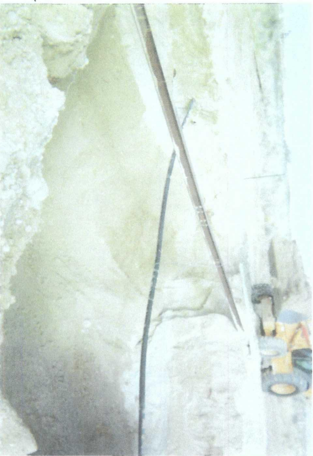
-backfilling excavation up to 6 ft BGS
