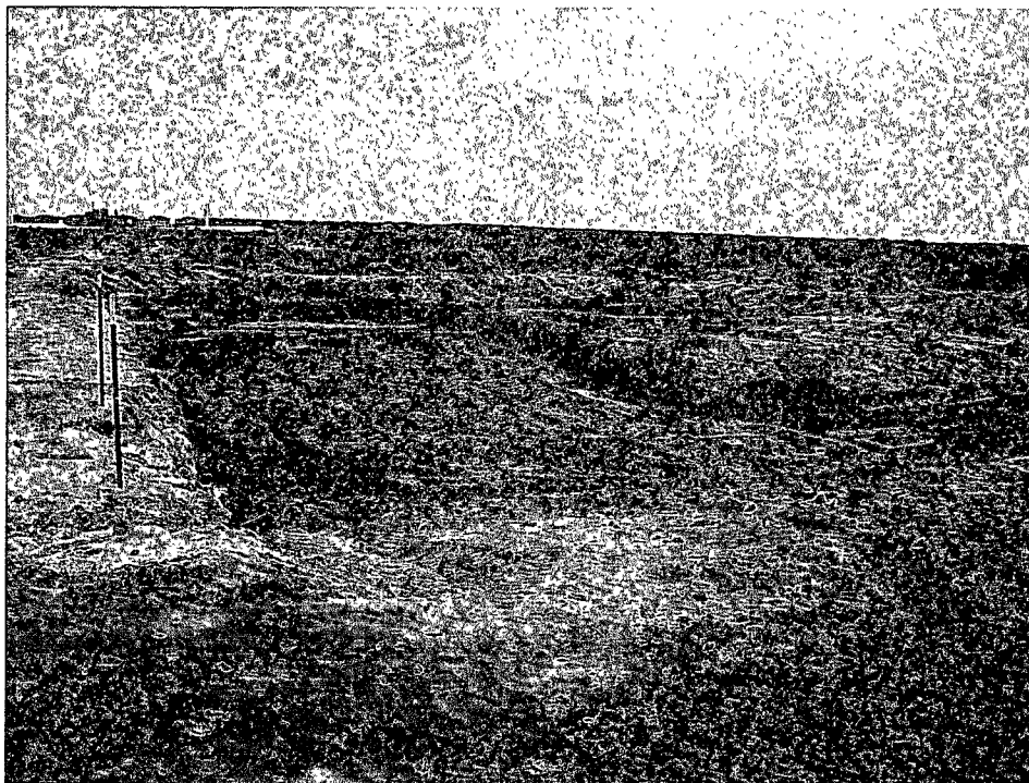
Site with clay liner in place.
