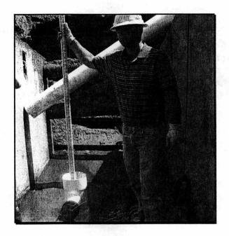
Tie-in of the 4" perforated pipe to the 8" vertical pipe
