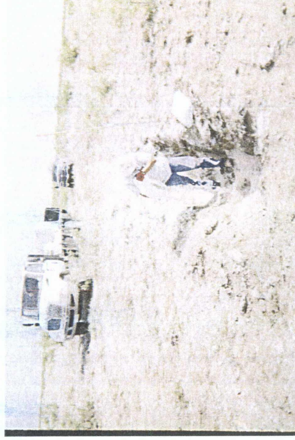
plugging SB #1 with bentonite
