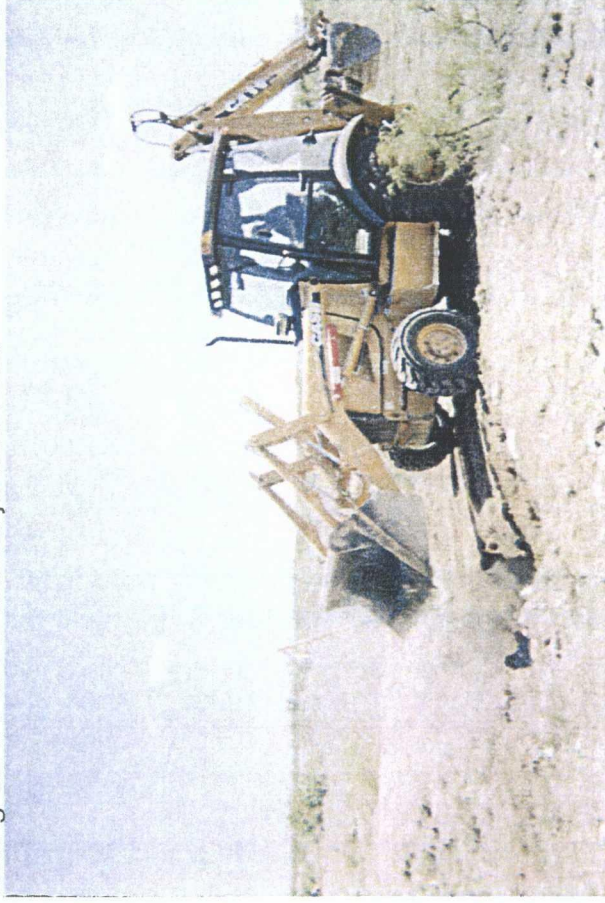
backfilling the former junction box site, facing northwest
