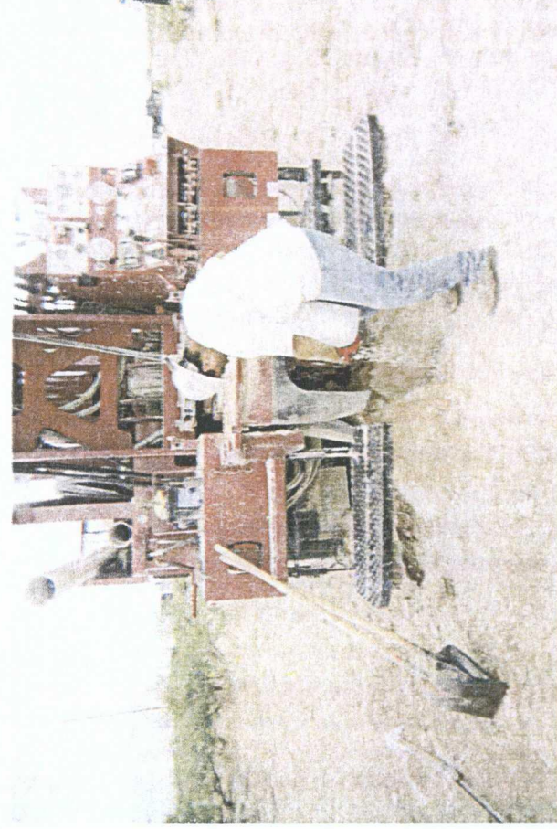
plugging SB #1 with bentonite
