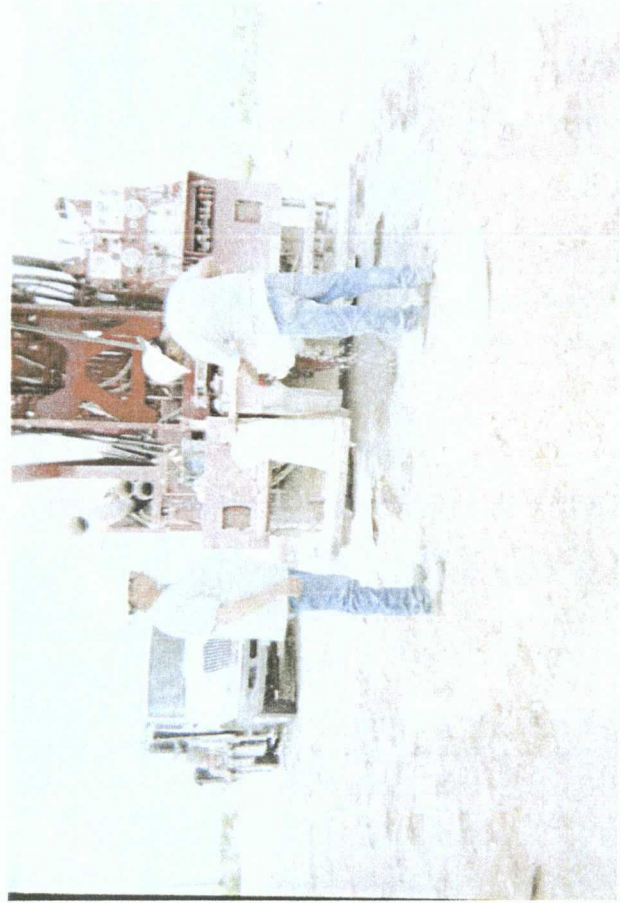
plugging SB #1 with bentonite
