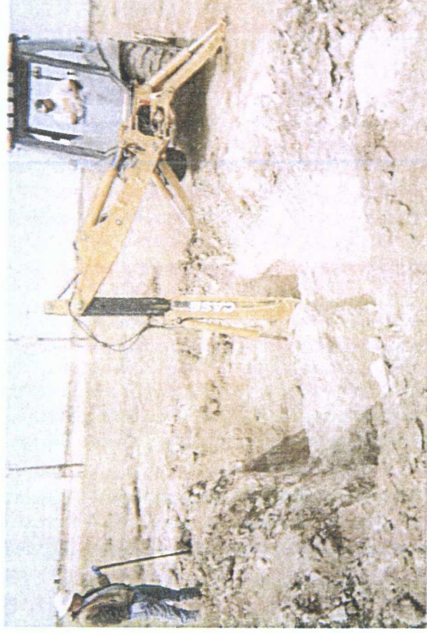
Delineation trench being excavated
