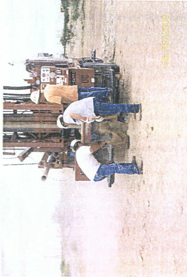
Drilling Soil Bore #1
