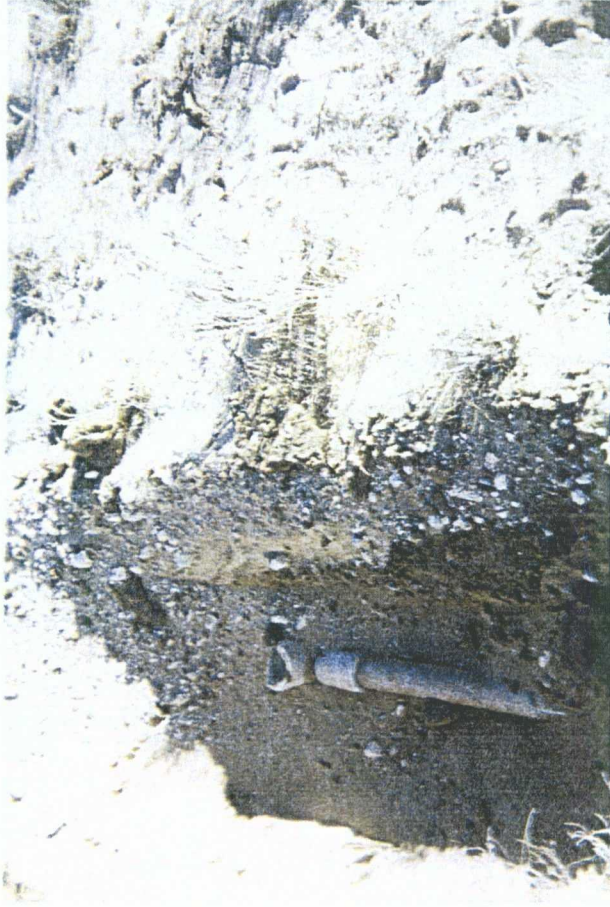
capped lines at former junction box, facing north
