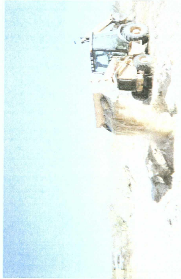
Backfilling excavation
