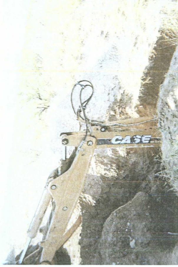
Delineation trench at former junction box
