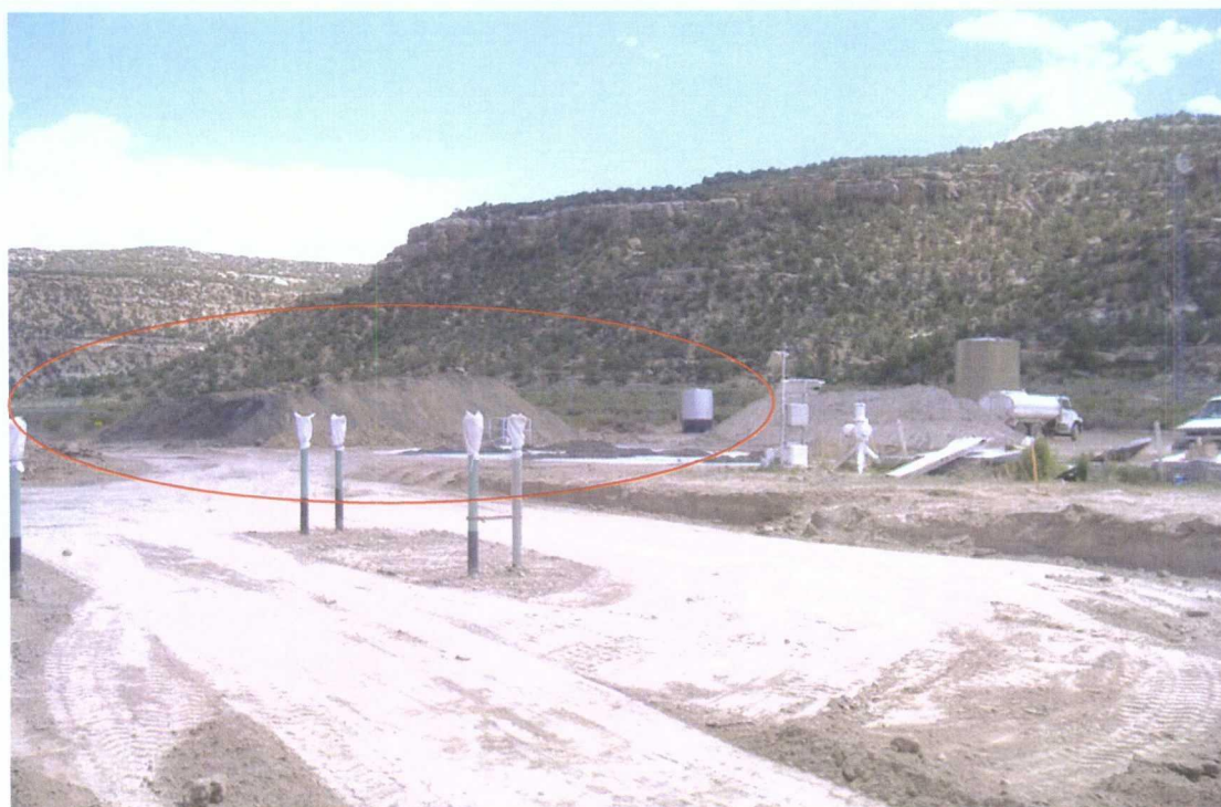
July 1, 2009 Photo 12: Stockpiles of contaminated soil removed from subsurface. Sample collected for analysis for disposal characterization (RCRA 8 Metals).
