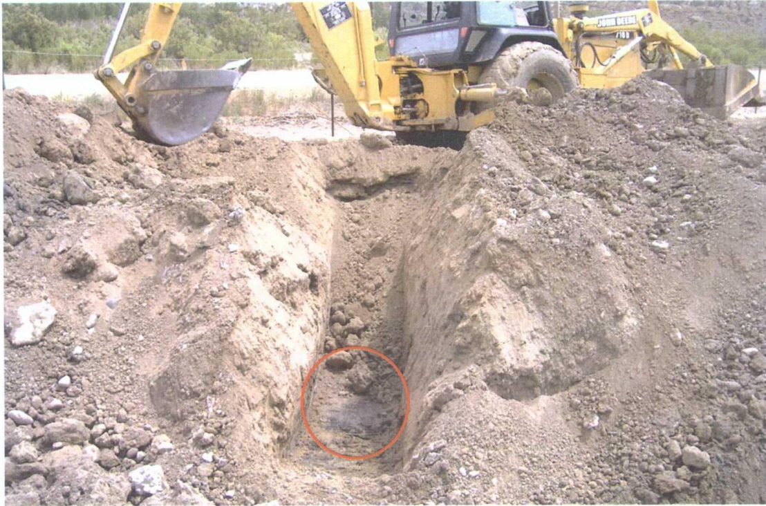
Photo 5: Contaminated soil encountered in pothole near fence/road (PH #4).
