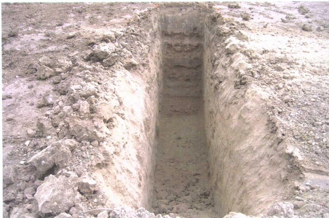
June 26, 2009 Photo 1: Example of clean overburden, approximately 6 feet deep.
