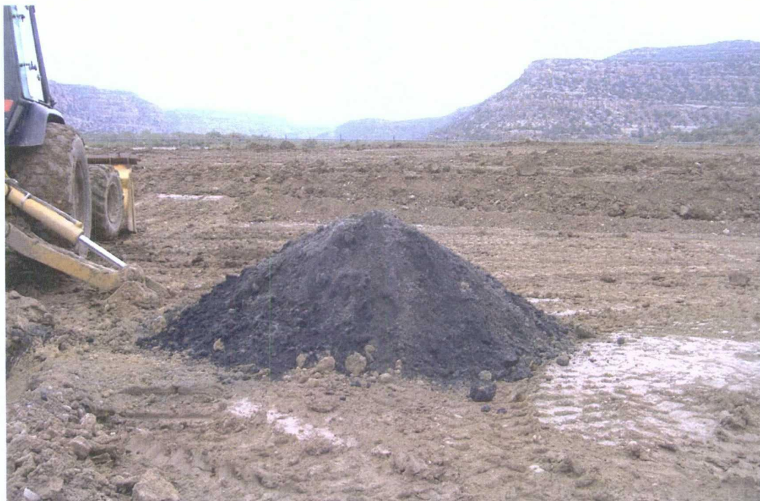
June 26, 3009 Photo 3: Contaminated soil removed from pothole (PH #1) dug on 6/26/2009.
