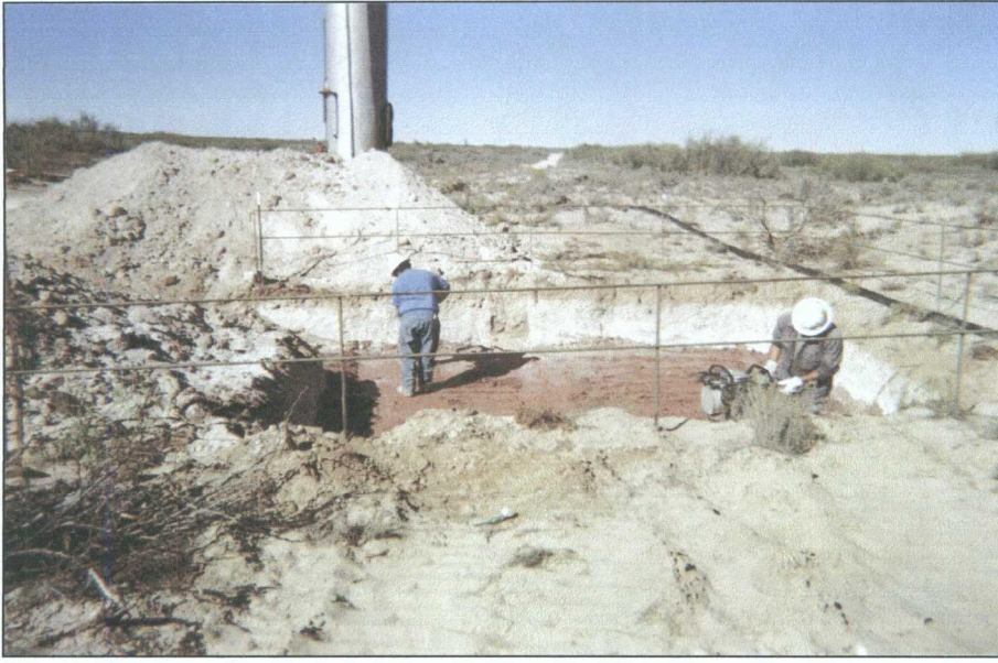
Figure 3 – Installation of a clay infiltration barrier following removal of the junction box at EMS State H EOL.
